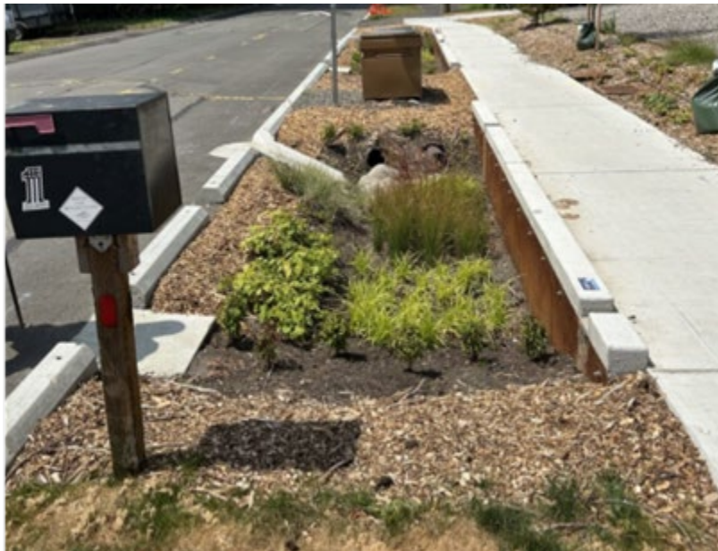
Figure 4-7. Constructed bioretention cell on the South Thornton NDS project
