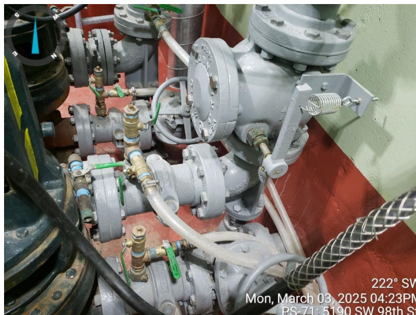
Figure 3-3. Completed Installation of New Piping and Valves at Pump Station 71
