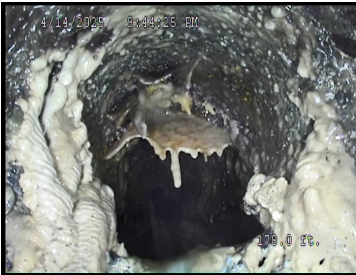
Figure 3-1. 2025 Mainline Image Demonstrating Visible FOG Accumulations from a Popular Fast Food Establishment Side Sewer Connection
