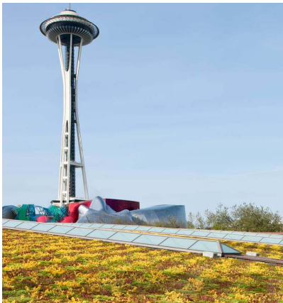
Seattle Center 5th Ave. N. Garage, designed by NBBJ/GGN; photo by Lara Swimmer
