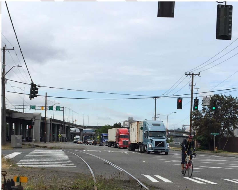
Existing conditions on East Marginal Way
