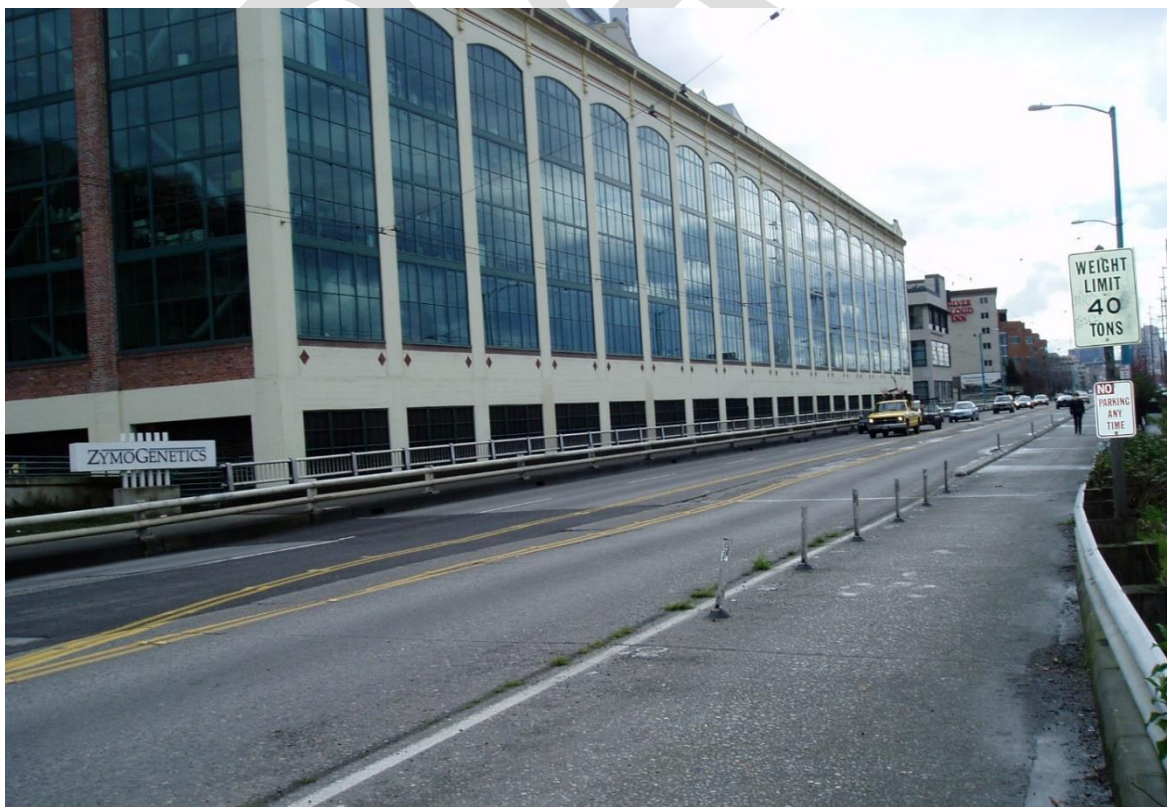
Existing conditions on Fairview Ave N
