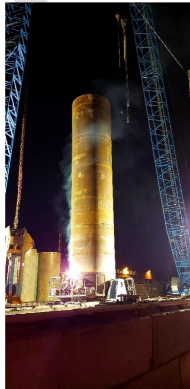
Crews weld shaft casing for Lander Bridge
