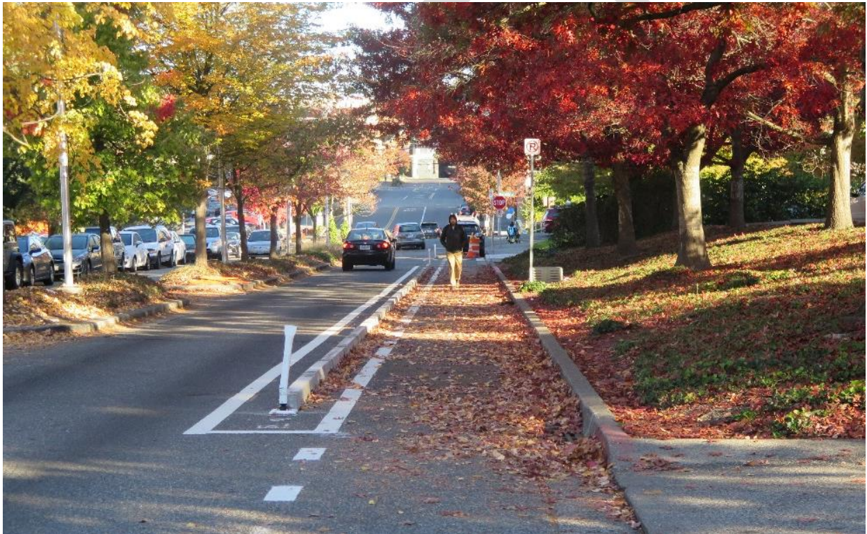
Low-cost sidewalk on 3rd Ave NE
