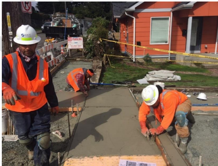
Crews building sidewalk
