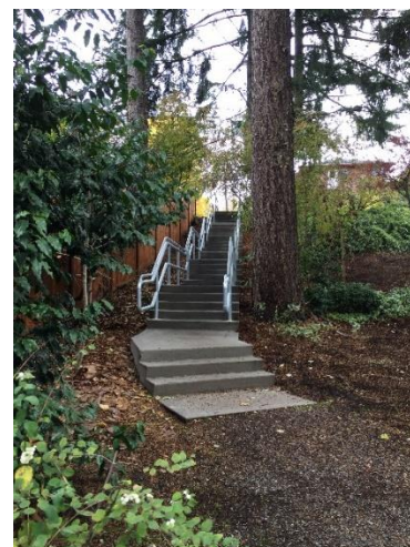
N 88th St stairway, after
