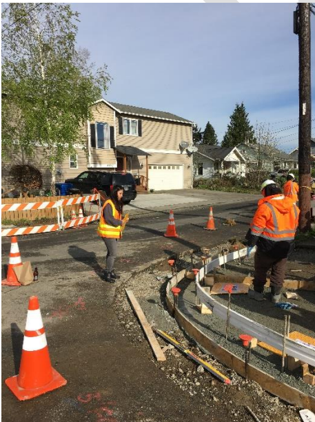
Forming new curb ramps and sidewalk corner
