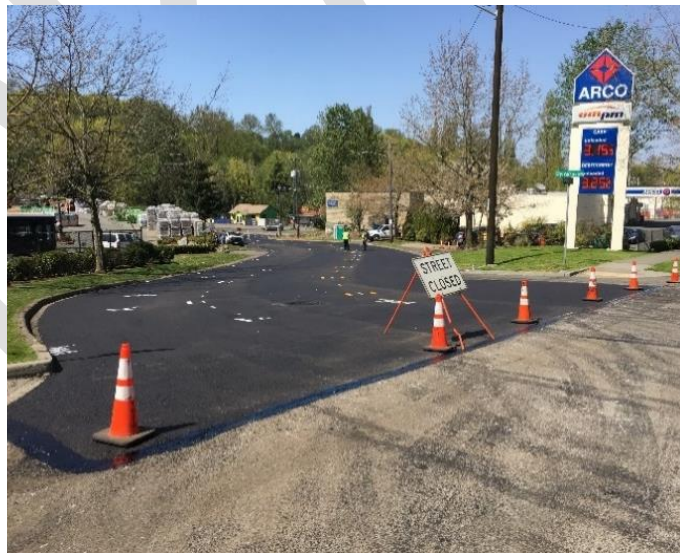
Pavement after repair
