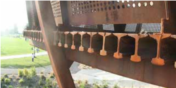
Reclaimed railroad rails, or other reclaimed materials, can become deck paving at the corner eddies.
