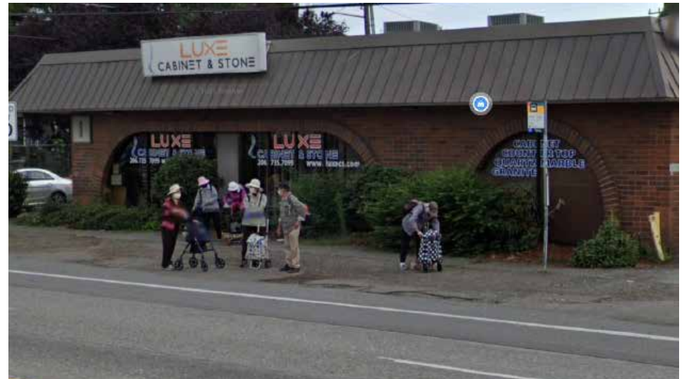
The existing north-bound 4th Ave S transit stop, just north of S Lucile St, requires bus drivers to pull onto broken paving or riders to traverse gravel to access buses.
