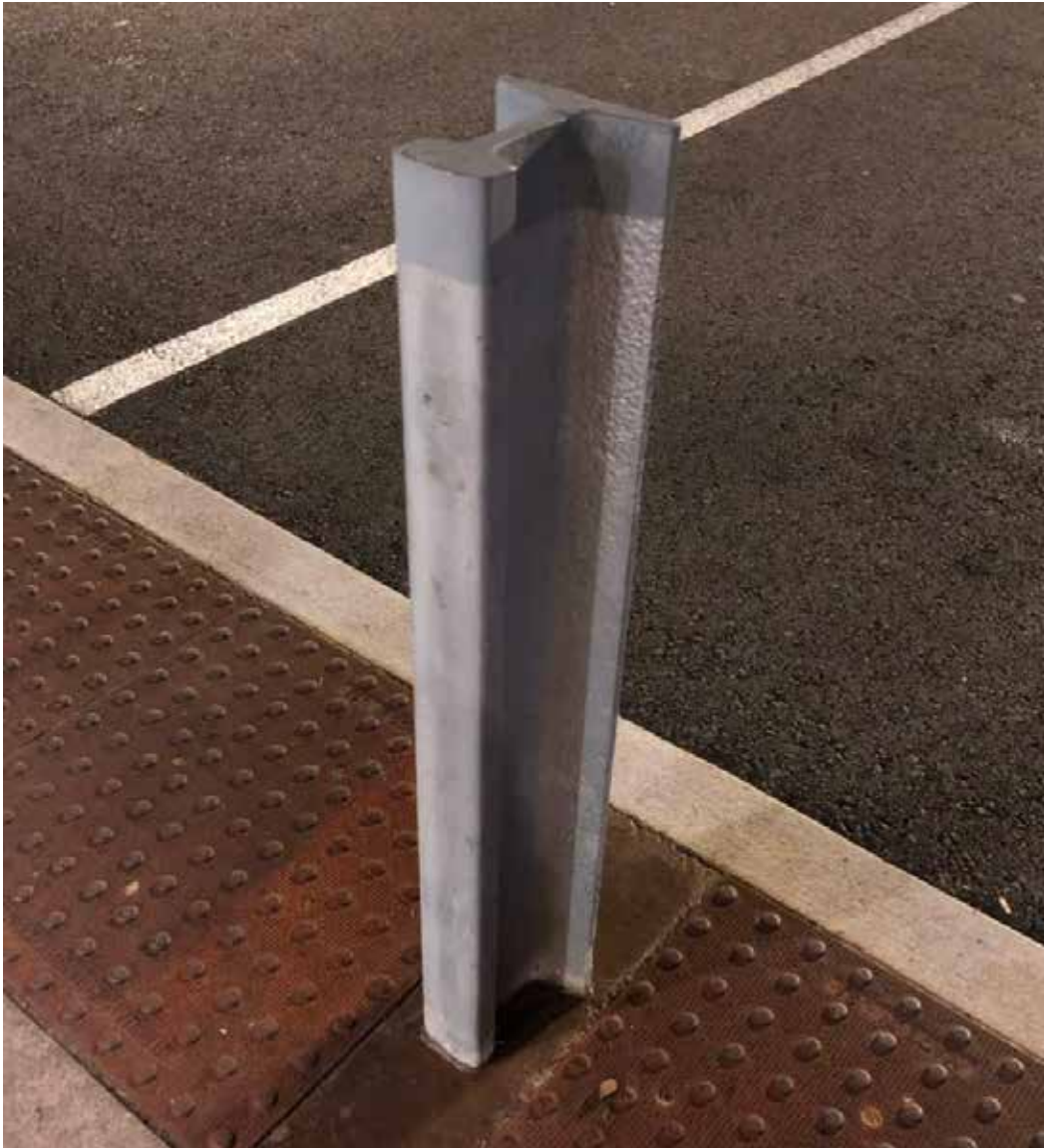
A reclaimed railroad rail at the former New Seasons Market in Ballard. In the case of the Georgetown Live-Work District, bollards such as this shall be set into yellow tactile warning strips whenever pedestrians might enter travel lanes. Image by Mark Ostrow.
