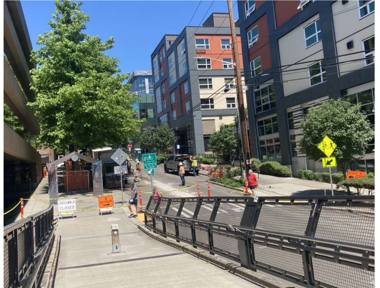
Thomas St Overpass, looking north onto 3 rd Ave W Ped & bike detour installed (6/2/21)
