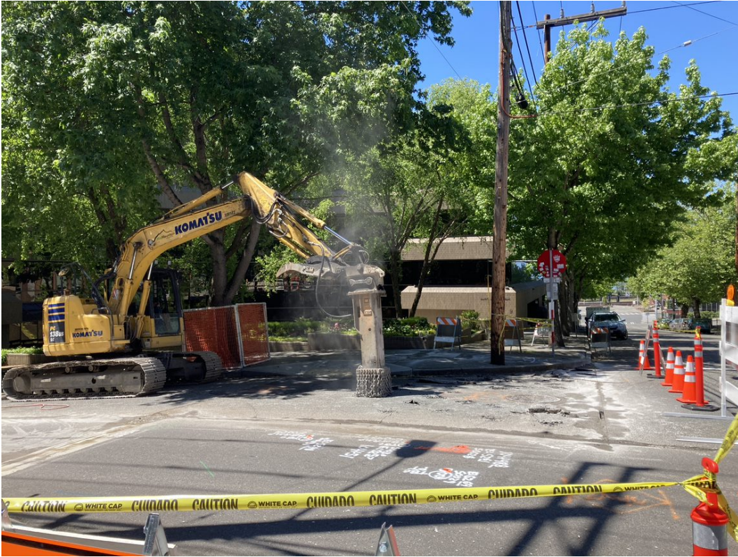
Demolition at 3 rd Ave W & Harrison St (6/2/21)
