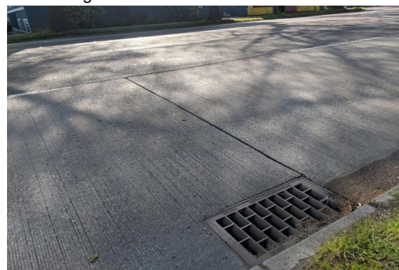
Figure 9.4 A typical storm drain along the Metro Route 7
