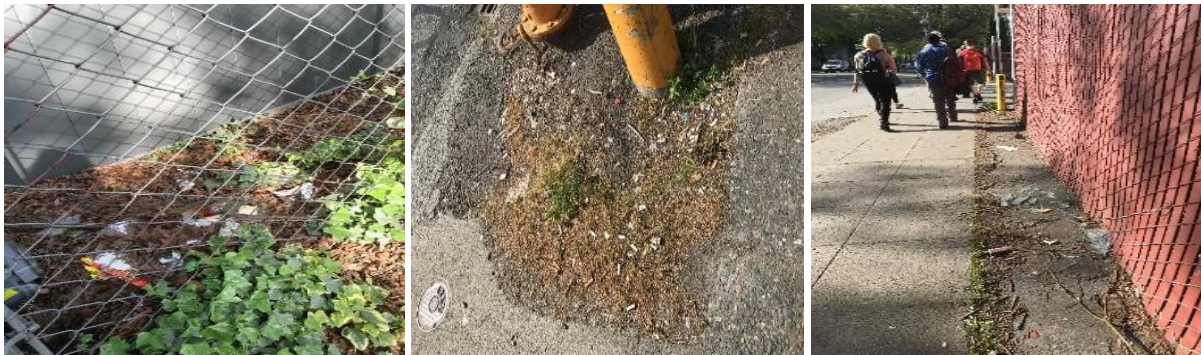
Figure 9.8 Pictures from May 3 rd , 2018 Site Visit depicting variety of litter currently present along Rainier Ave S
