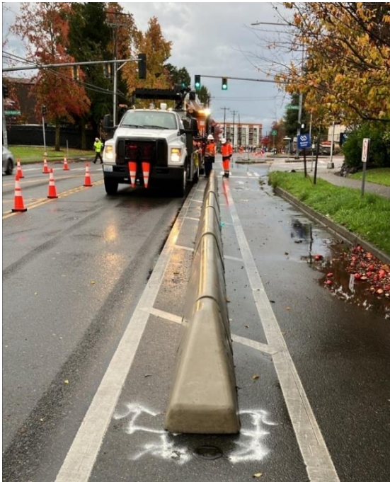
Toronto-style barrier being installed in Seattle
