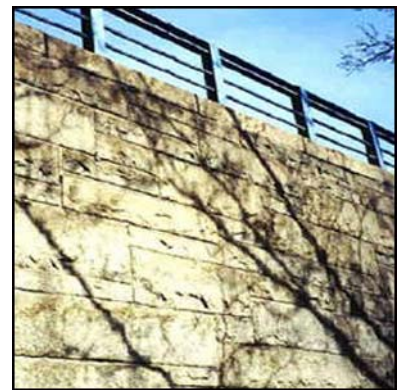
"Textured concrete wall - using form liner
