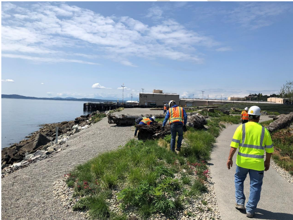
Figure A-8 Elliott Bay Trail Improvements Underway near Expedia's Campus, Summer 2019
