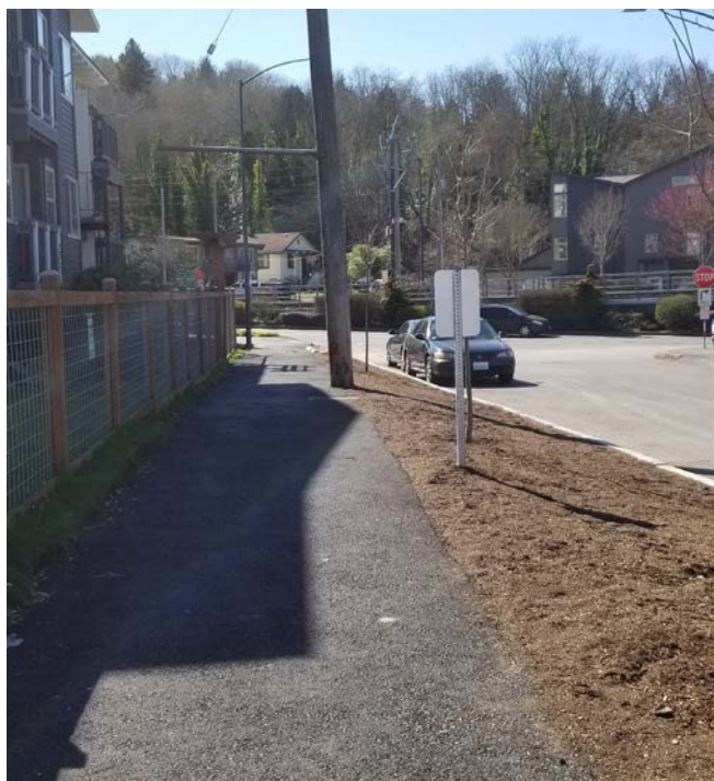
Cost-effective asphalt walkway on S Byron St
