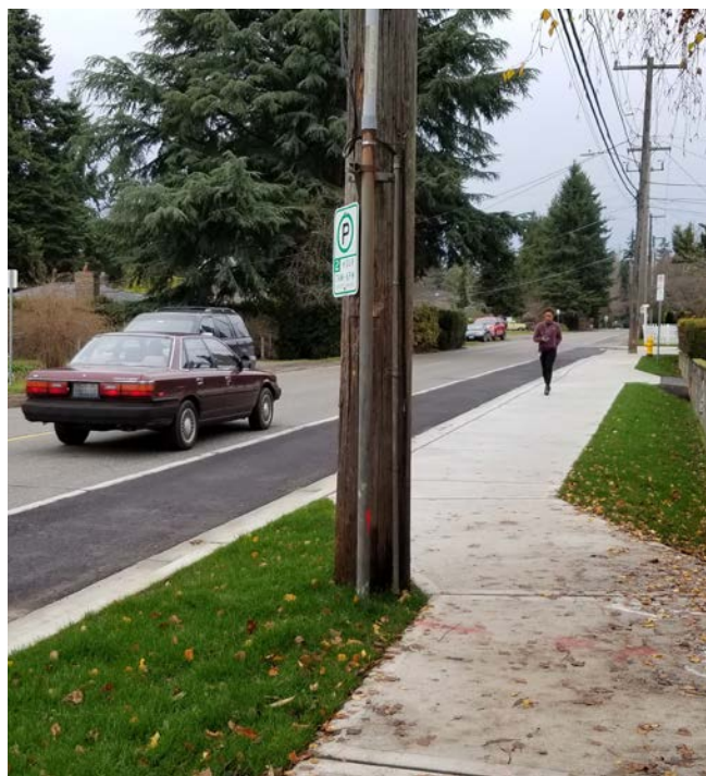
New traditional sidewalk on Meridian Ave N
