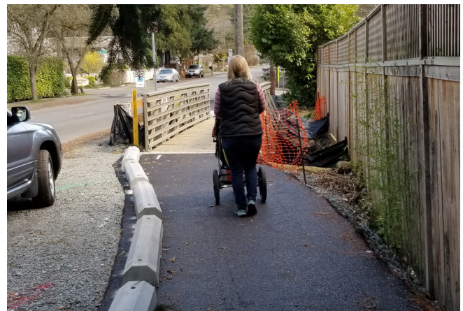
Delineated, at-grade asphalt walkways
