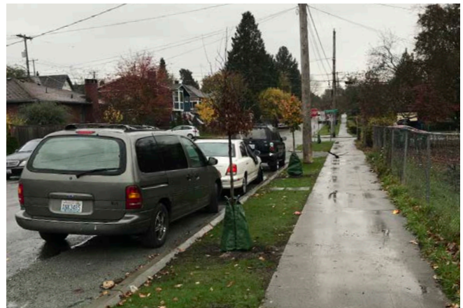
Delineated, at-grade concrete walkways
