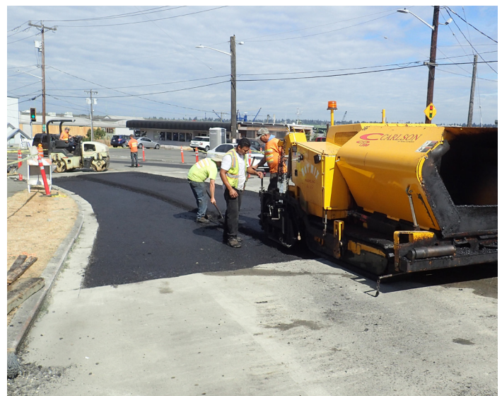
An example of crews paving
