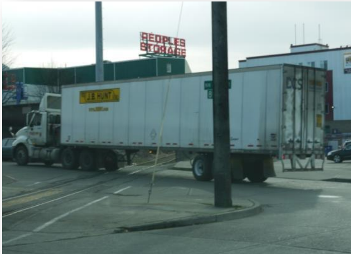
Utility pole placed close to an intersection. Transpo Group.
