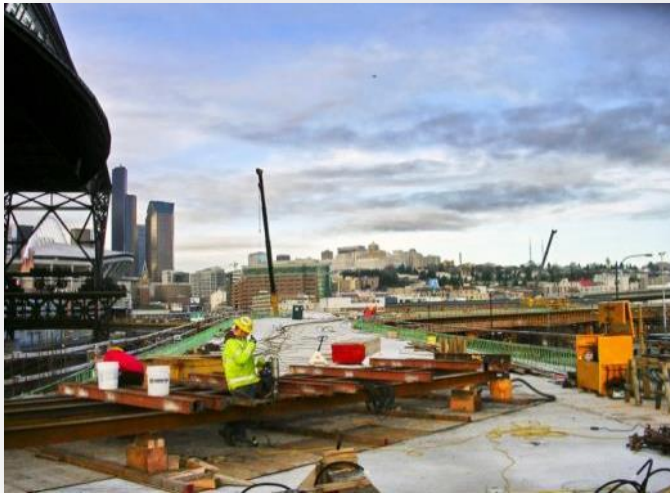
SR 519 under construction. WSDOT.
