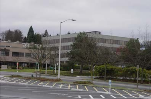
Looking south across NE 100th Street from Northgate south lot
