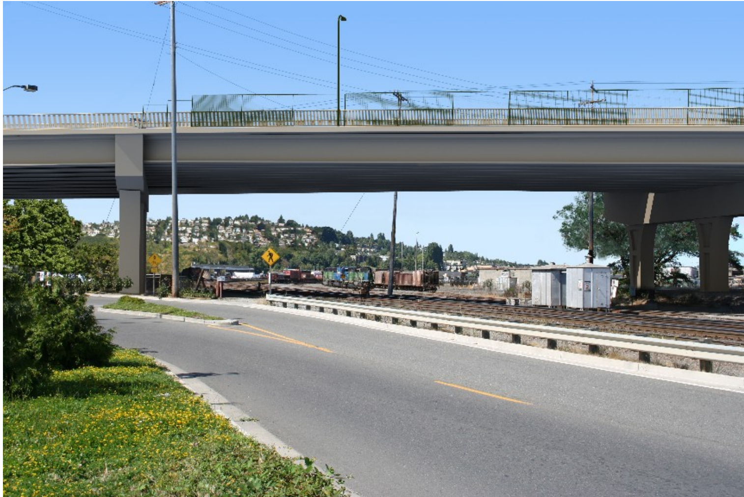
Figure 64 PRESTRESSED CONCRETE GIRDERS (looking north from Alaskan Way West)
