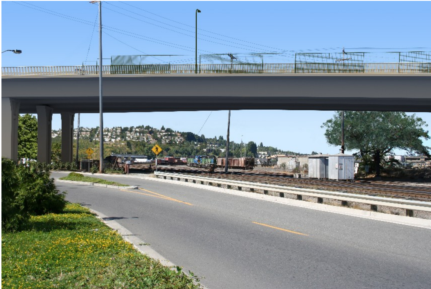
Figure 65 STRAIGHT CAST-IN-PLACE CONCRETE BOX GIRDER (looking north from Alaskan Way West)
