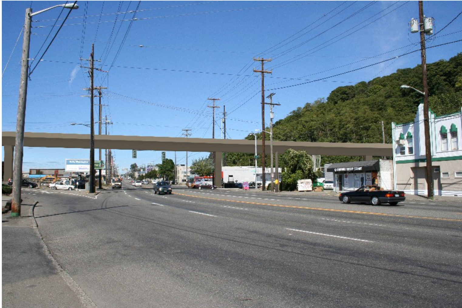
Figure 62 STRAIGHT CAST-IN-PLACE CONCRETE BOX GIRDER (looking north on 15 th Avenue West)
