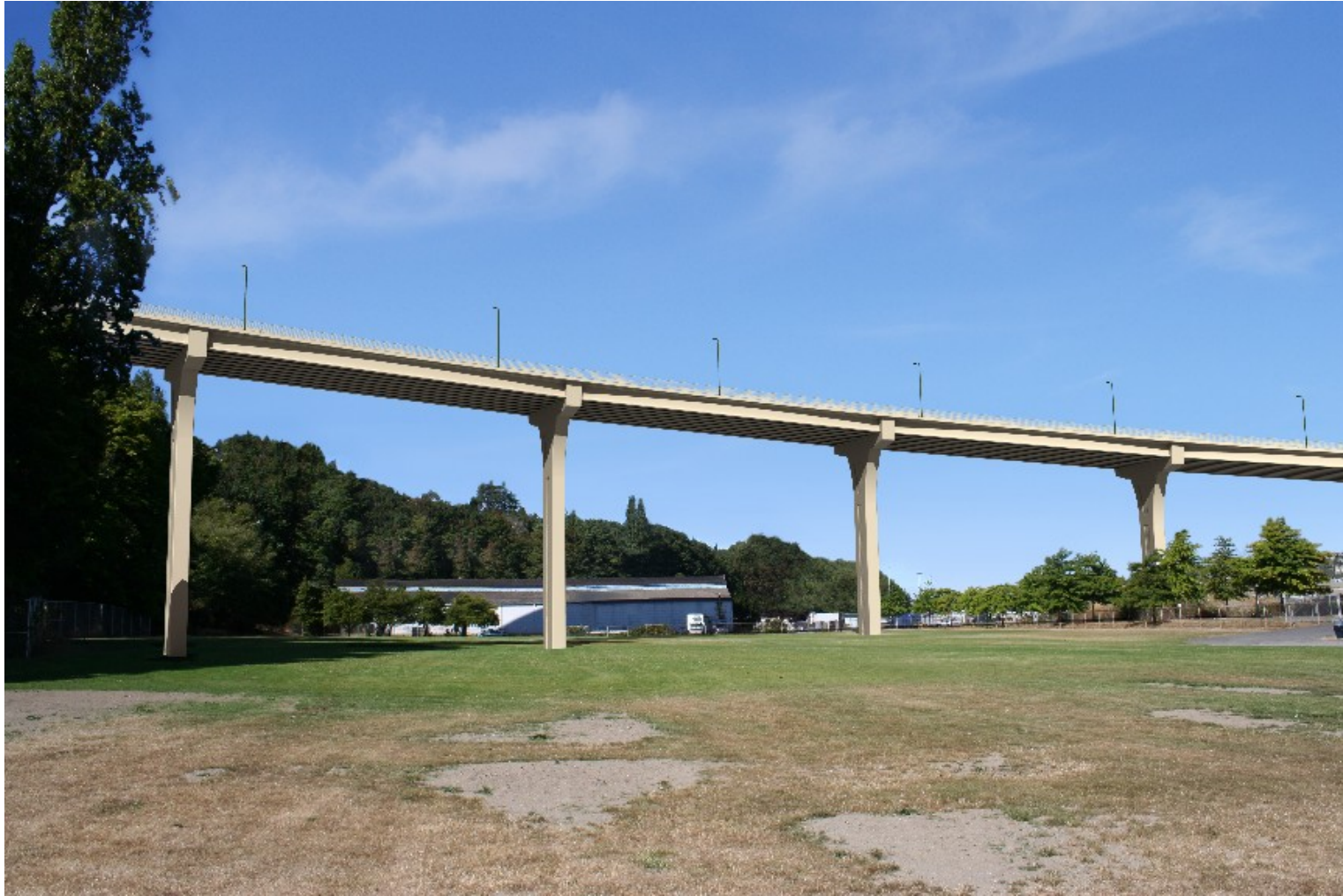
Figure 70 PRESTRESSED CONCRETE GIRDERS (looking north in Smith Cove Acquisition park site)
