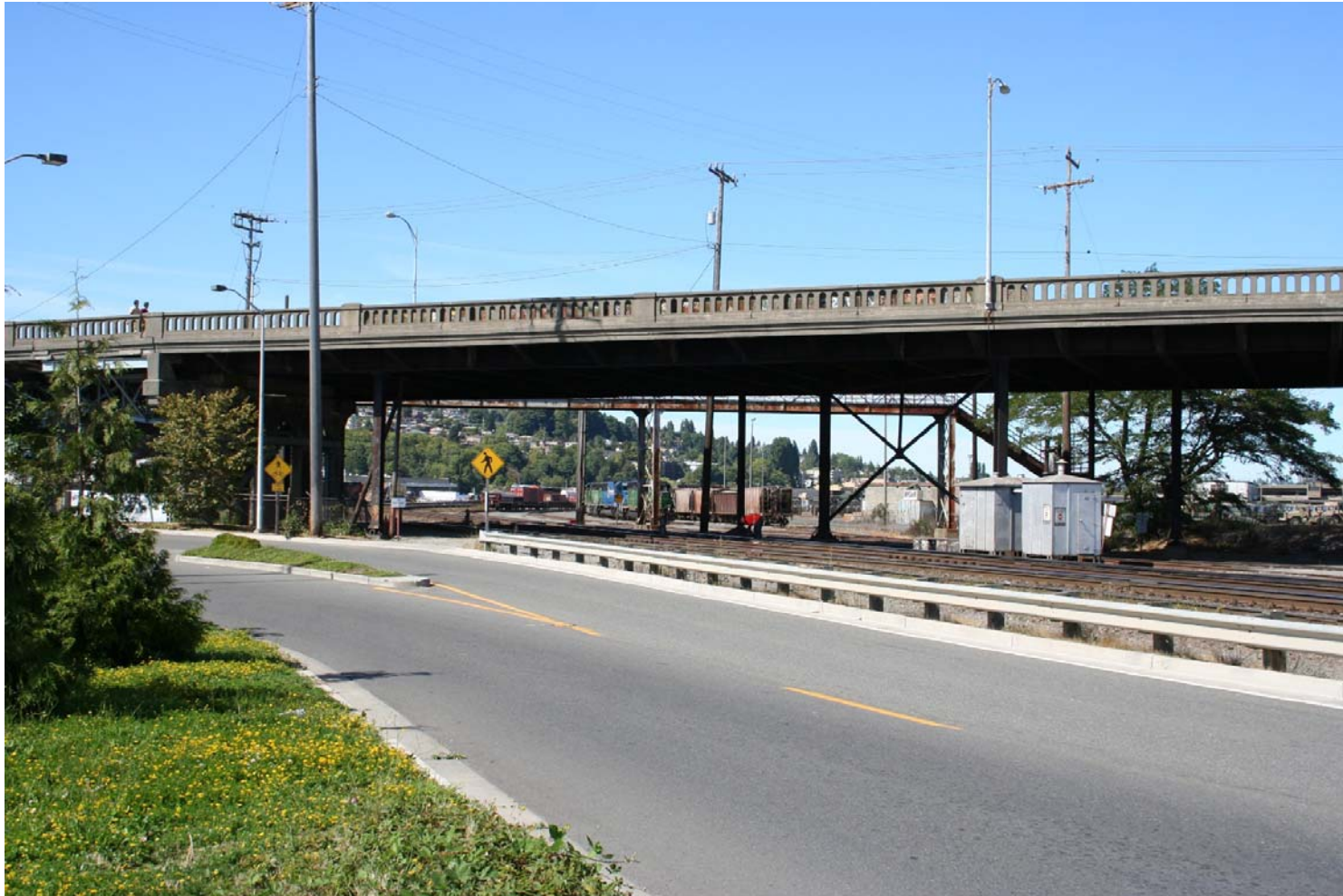
Figure 63 EXISTING BRIDGE (looking north from Alaskan Way West)
