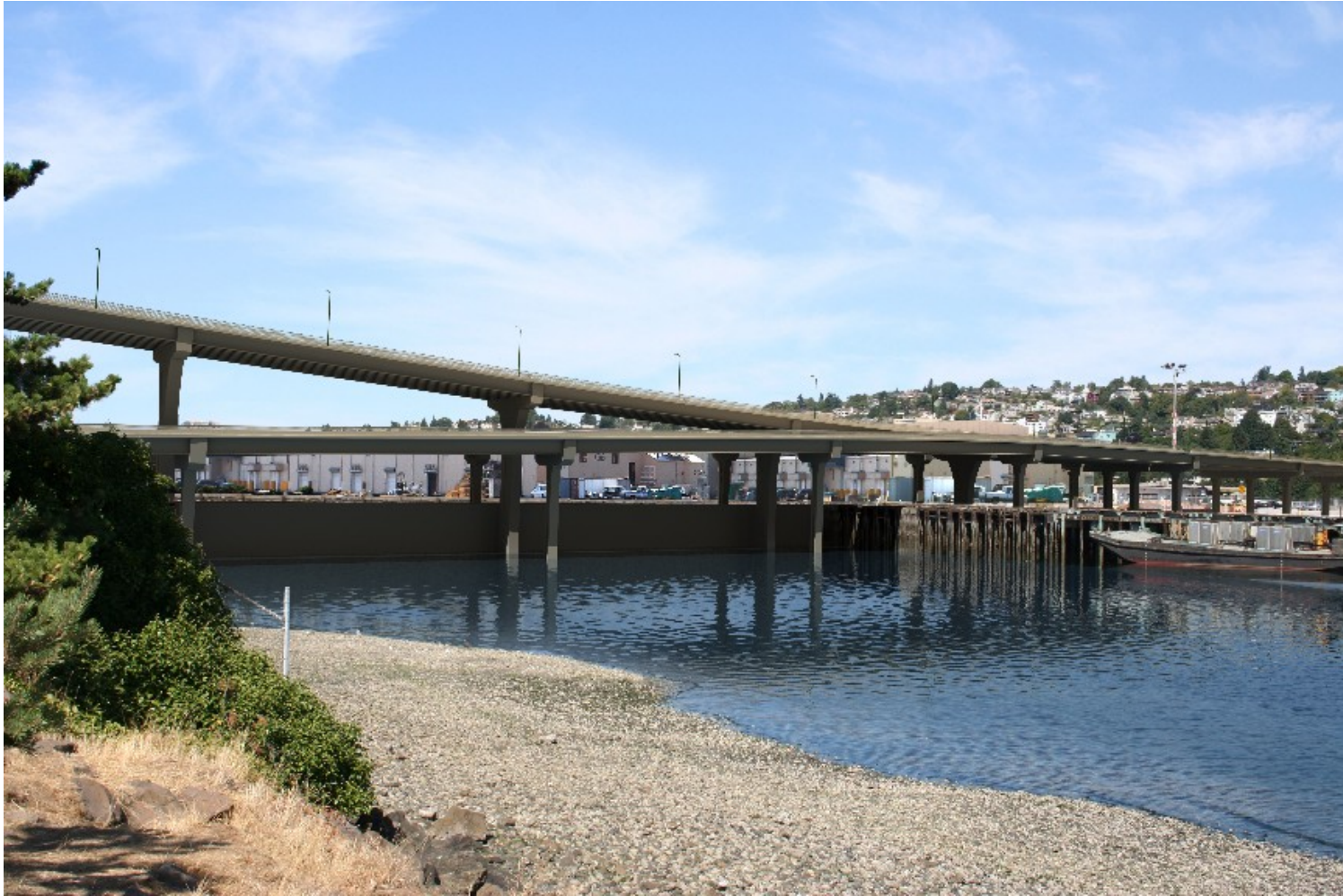
Figure 67 PRESTRESSED CONCRETE GIRDERS (looking northeast from Smith Cove Park)
