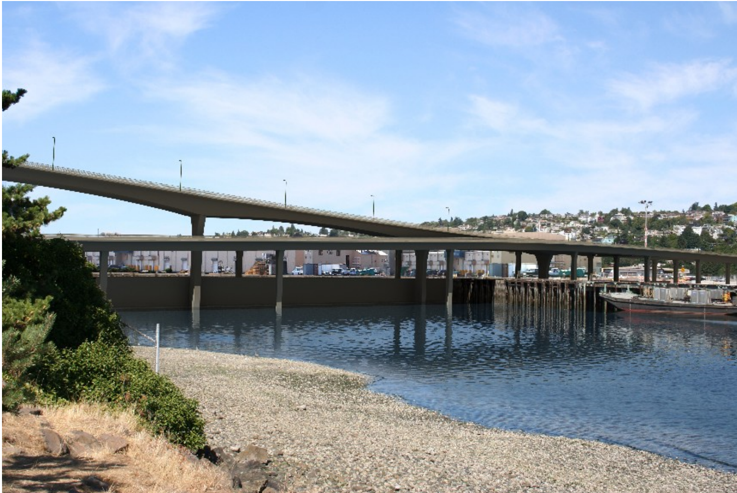
Figure 68 HAUNCHED CAST-IN-PLACE CONCRETE BOX GIRDER (MAINLINE STRUCTURE) STRAIGHT CAST-IN-PLACE CONCRETE BOX GIRDER (23 rd AVENUE RAMPS STRUCTURE)
