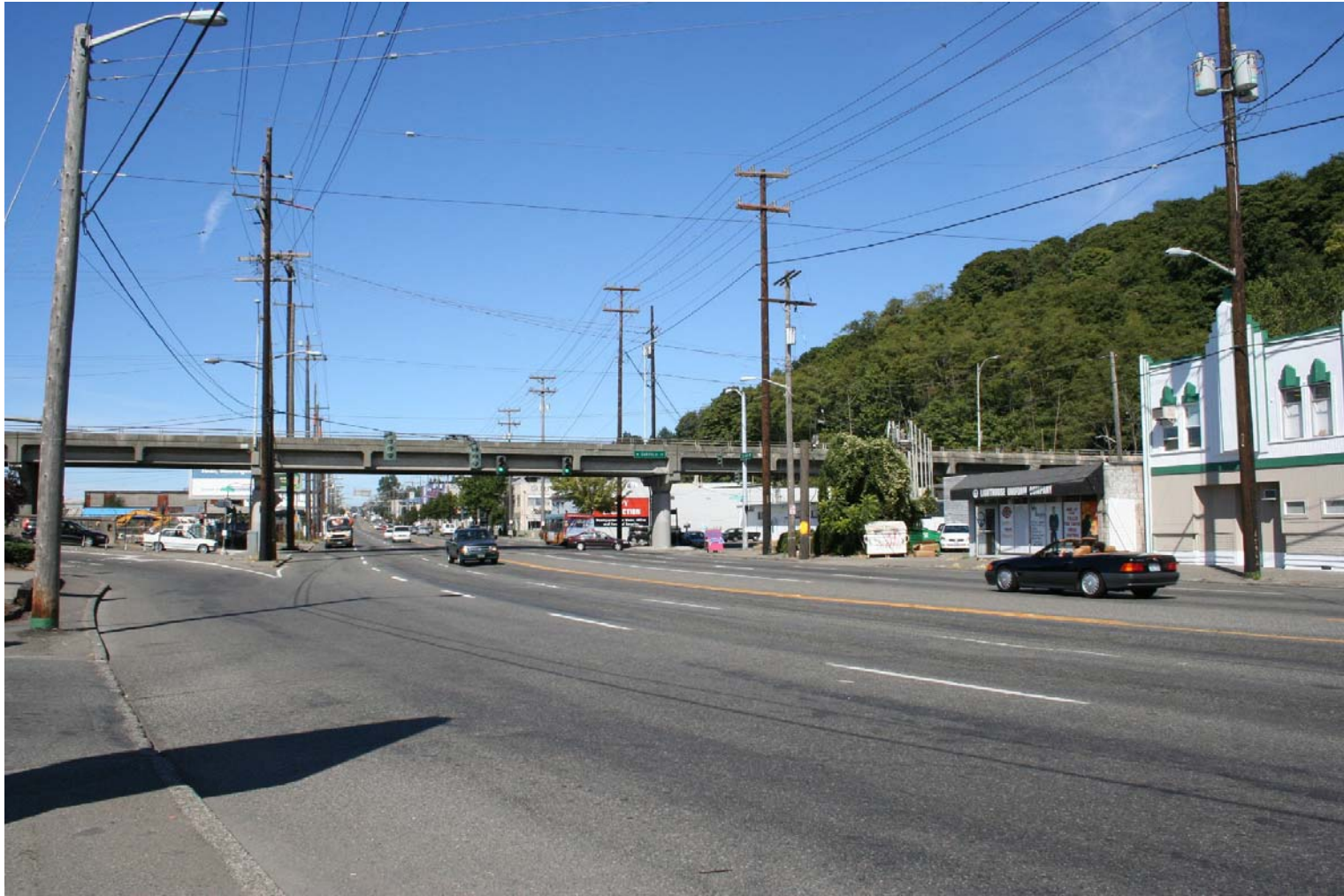
Figure 59 EXISTING BRIDGE (looking north on 15 th Avenue West)
