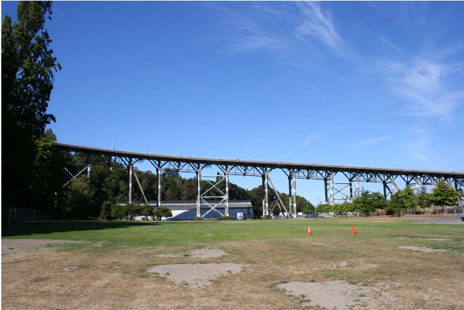
Figure 69 EXISTING BRIDGE (looking north in Smith Cove Acquisition park site)
