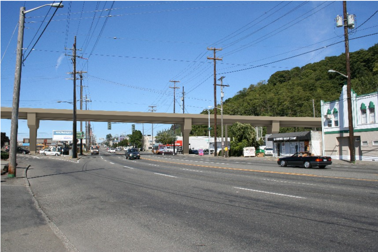
Figure 60 PRESTRESSED CONCRETE GIRDERS (looking north on 15 th Avenue West)
