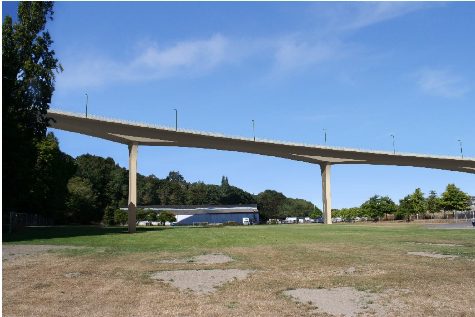
Figure 71 HAUNCHED CAST-IN-PLACE CONCRETE BOX GIRDER (looking north in Smith Cove Acquisition park site)
