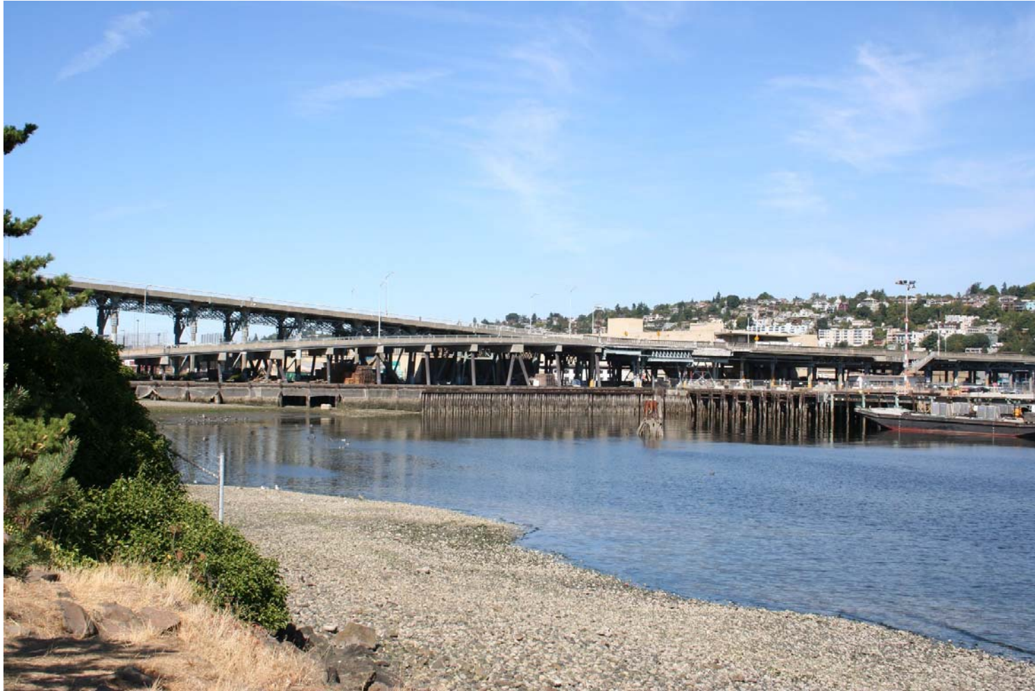
Figure 66 EXISTING BRIDGE (looking northwest from Smith Cove Park)
