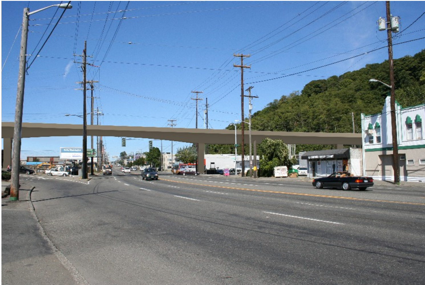
Figure 61 HAUNCHED CAST-IN-PLACE CONCRETE BOX GIRDER (looking north on 15 th Avenue West)
