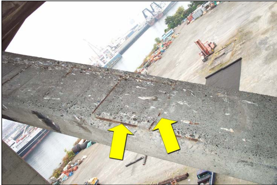
Figure 19 - Bents 64 to 65: Station 25+58 to 26+18 (Reference Photograph 80)
