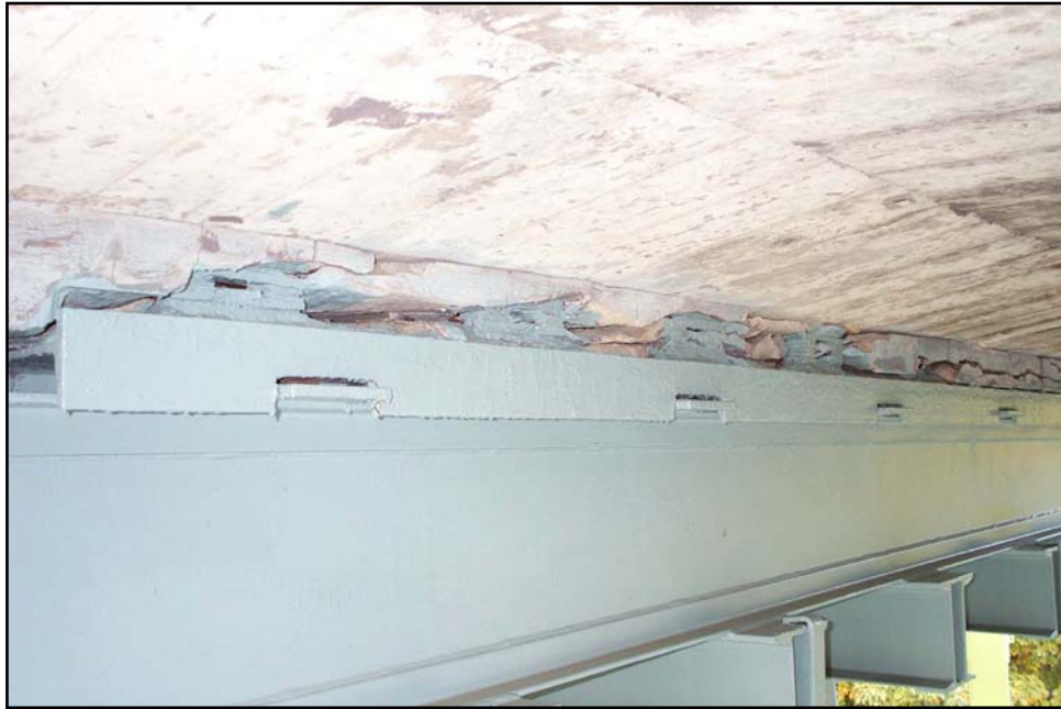
Figure 25 - Bent 73: Station 30+30 (Reference Photograph 91)
