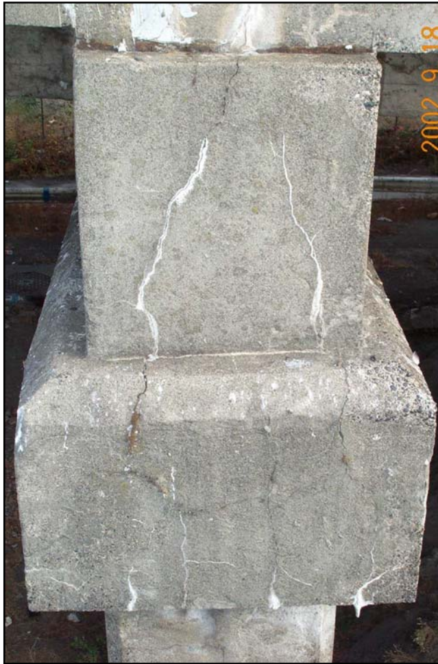
Figure 4 - Bent 4: Station 4+77 (Reference Photograph 11)
