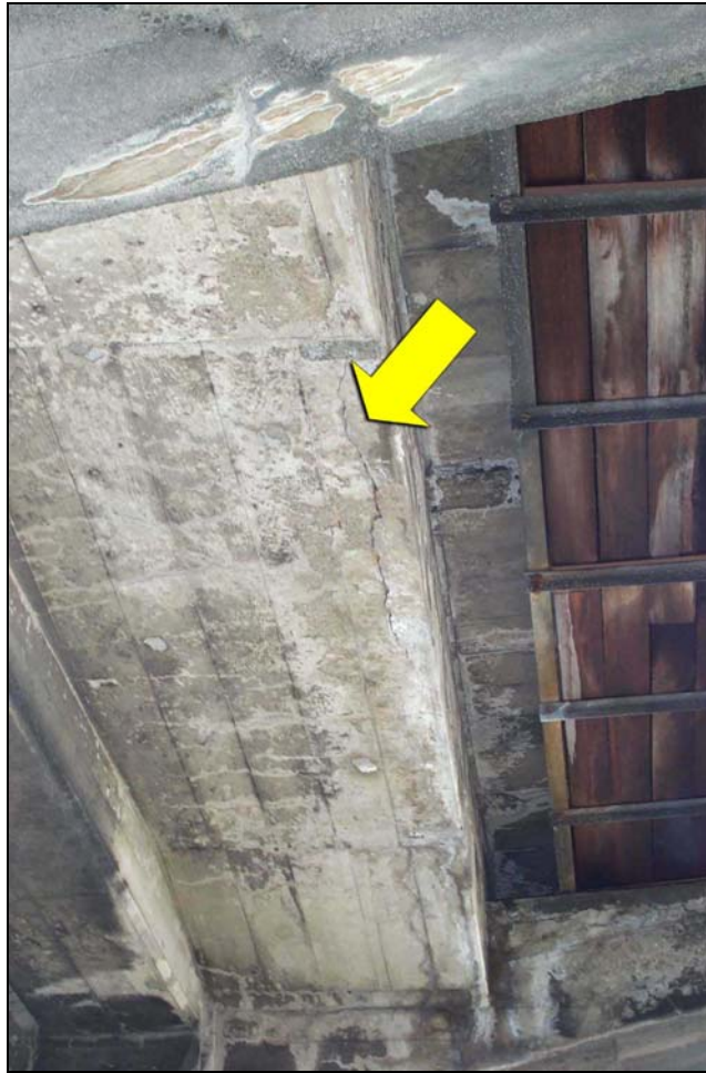
Figure 21 - Bents 70 to 71: Station 28+67 to 29+27 (Reference Photograph 85)
