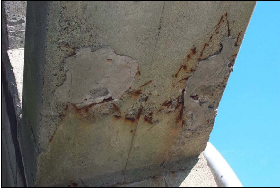
Figure 23 - Bents 72 to 73: Station 29+70 to 30+30 (Reference Photograph 93)
