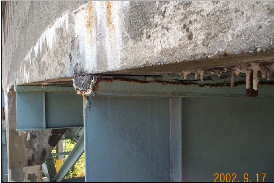
Figure 13 - Bents 30 to 31: Station 13+32 to 13+68 (Reference Photograph 52)
