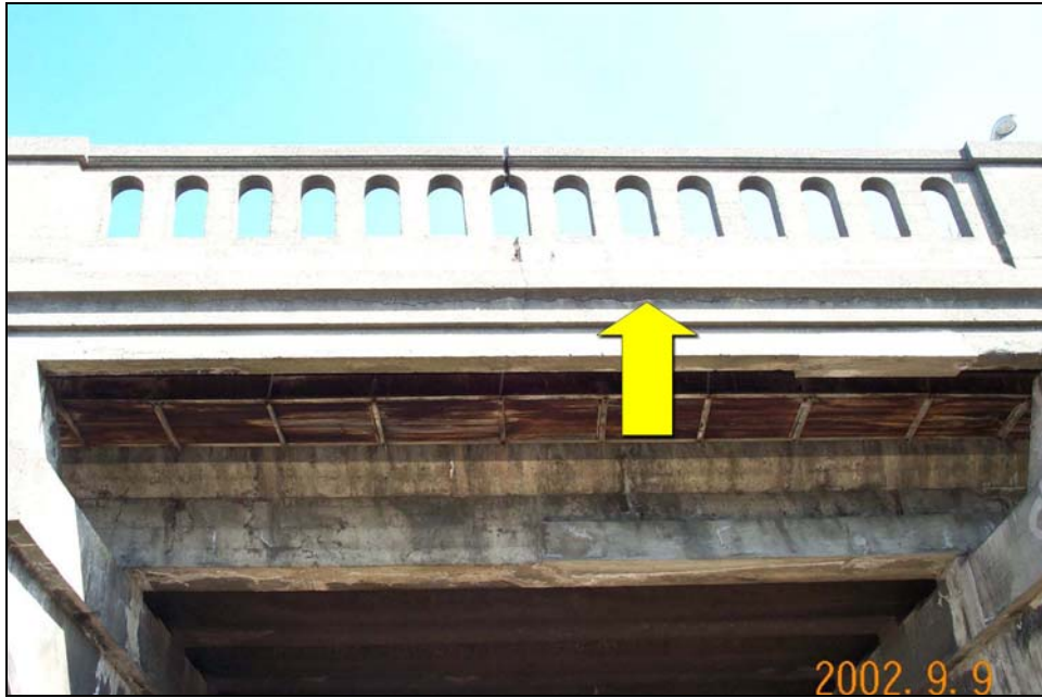
Figure 2 - Bents 2 to 3: Station 4+29 to 4+53 (Reference Photograph 8)
