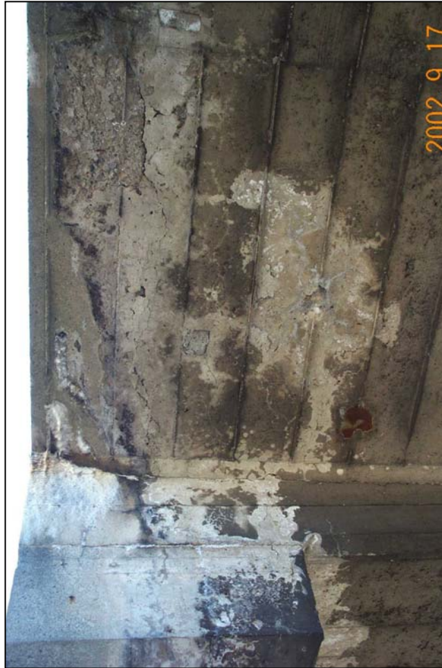
Figure 10 - Bent 23: Station 11+00 (Reference Photograph 44)
