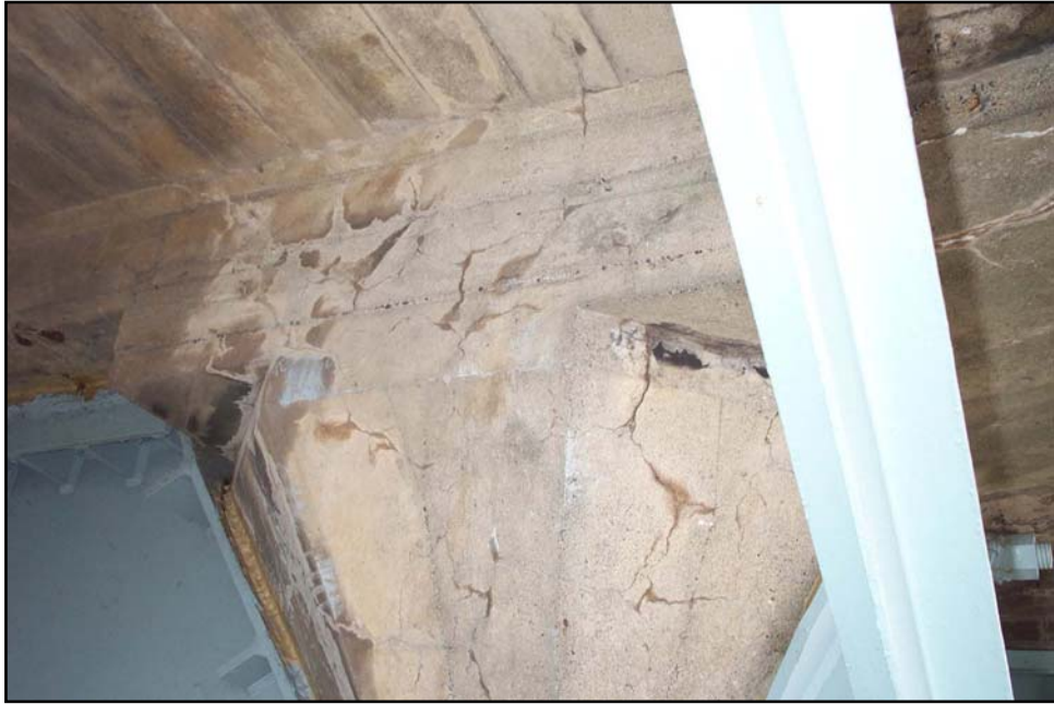
Figure 17 - Bent 53: Station 20+95 (Reference Photograph 73)
