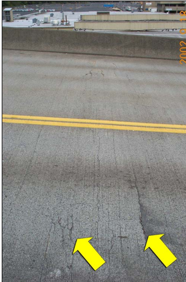
Figure 28 - Bent 48 Station 19+31 (Reference Photograph 108)
