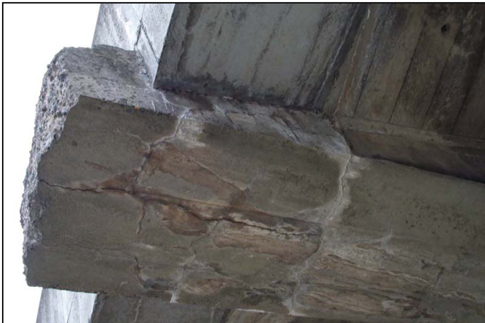
Figure 18 - Bents 64 to 65: Station 25+58 to 26+18 (Reference Photograph 76)
