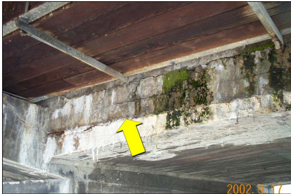
Figure 11 - Bent 24: Station 11+32 (Reference Photograph 46)
