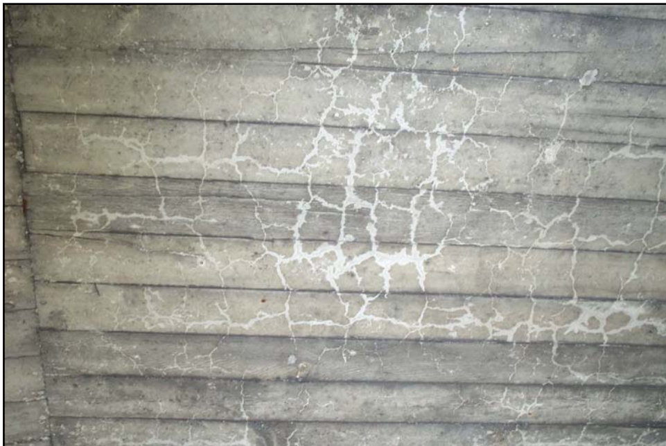
Figure 26 - Bents 74 to 75: Station 30+73 to 31+33 (Reference Photograph 97)
