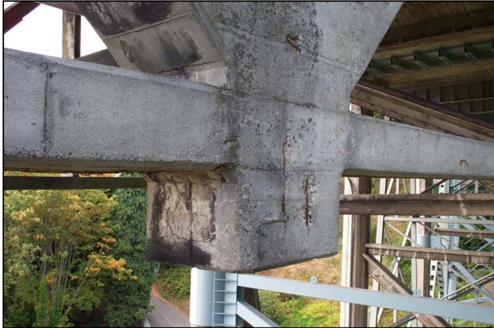
Figure 27 - Bents 74 to 75: Station 30+73 to 31+33 (Reference Photograph 99)
