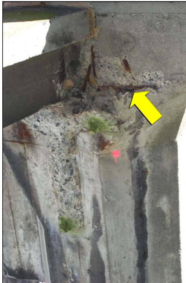
Figure 22 - Bent 72: Station 29+70 (Reference Photograph 90)
