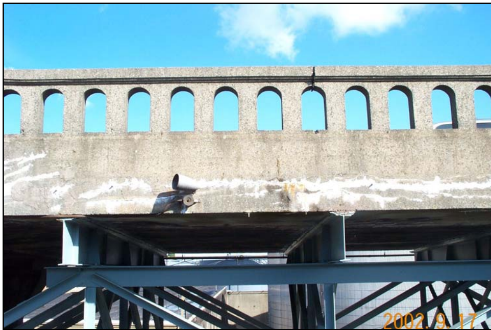
Figure 12 - Bents 30 to 31: Station 13+32 to 13+68 (Reference Photograph 51)
