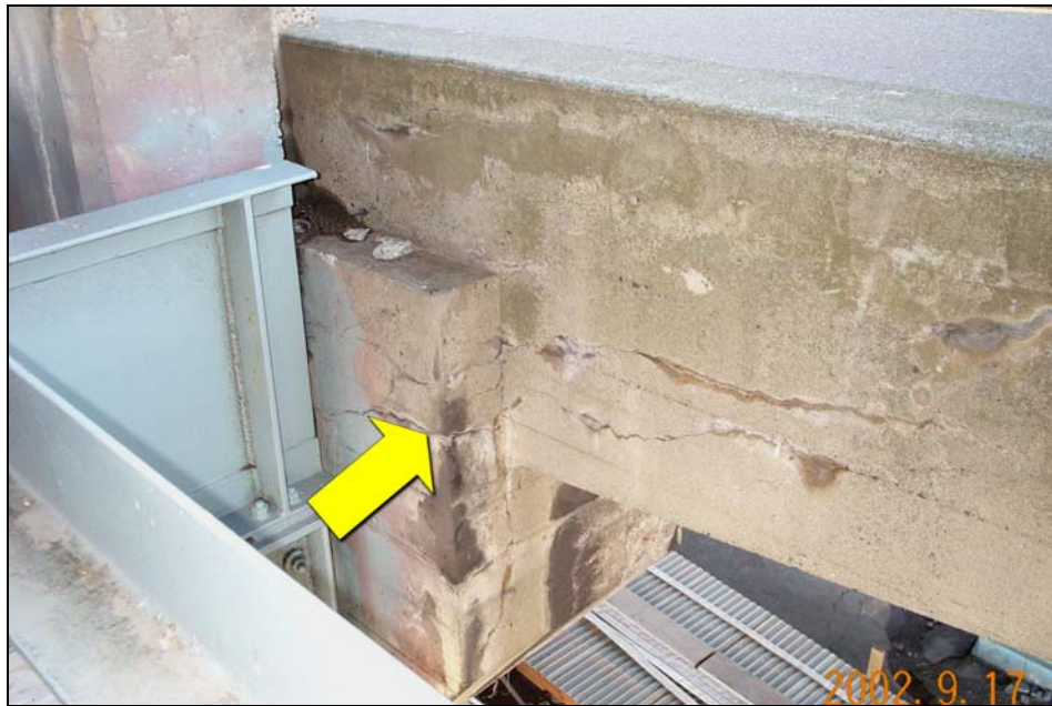
Figure 9 - Bent 24: Station 11+32 (Reference Photograph 41)
