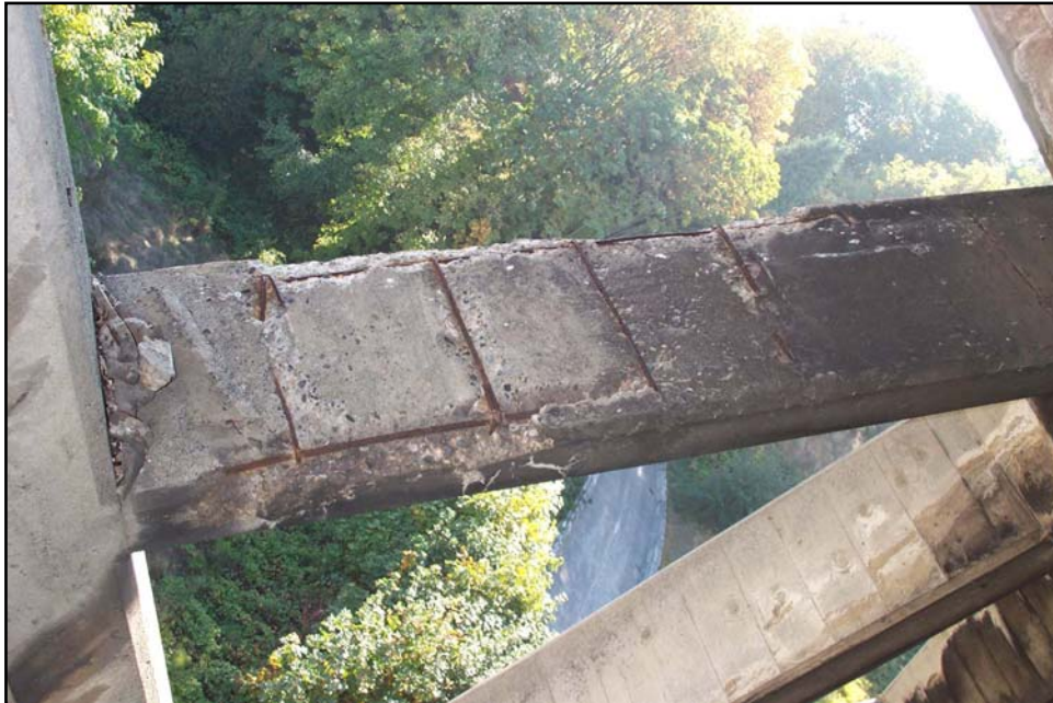
Figure 24 - Bents 72 to 73: Station 29+70 to 30+30 (Reference Photograph 94)
