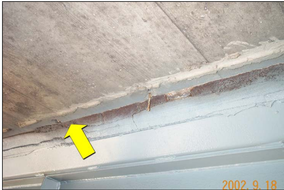
Figure 7 - Bents 16 to 17: Station 8+70.45 to 9+03.15 (Reference Photograph 27)
