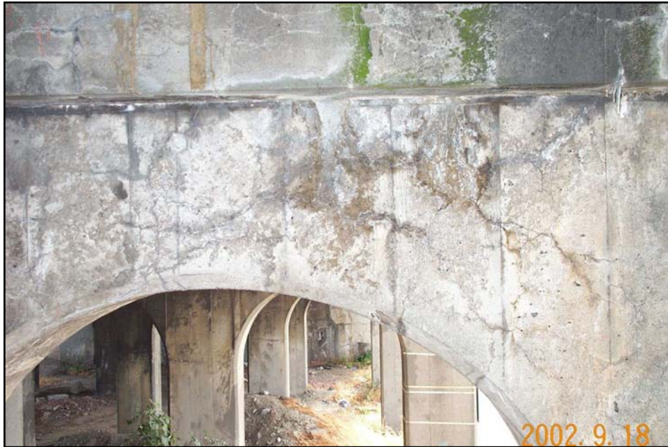
Figure 5 - Bent 4: Station 4+77 (Reference Photograph 17)
