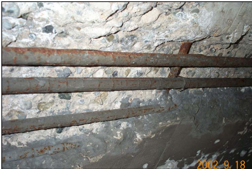
Figure 16 - Bents 41 to 42 Station 17+07 to 17+39.50 (Reference Photograph 67)
