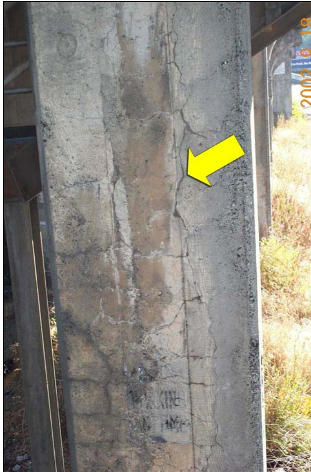
Figure 6 - Bent 5: Station 5+01 (Reference Photograph 22)
