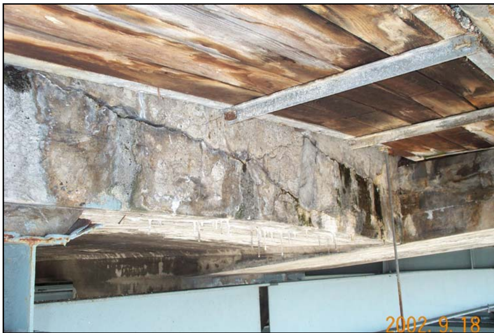
Figure 14 - Bents 41 to 42: Station 17+07 to 17+39.50 (Reference Photograph 61)
