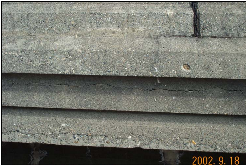
Figure 3 - Bent 4: Station 4+77 (Reference Photograph 9)
