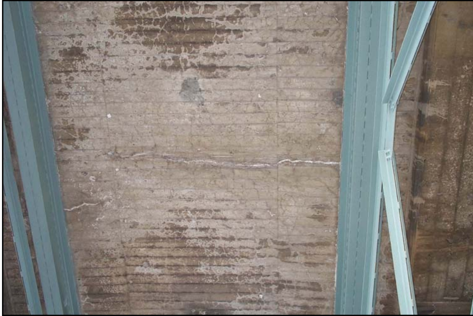
Figure 29 - Bent 48 Station 19+31 (Reference Photograph 109)
