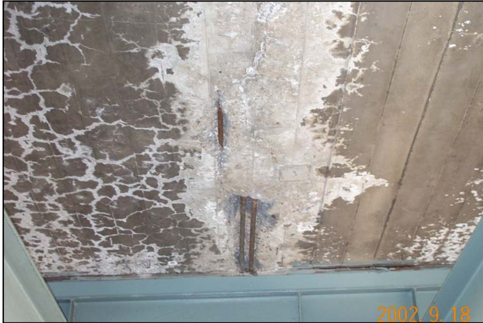
Figure 15 - Bents 41 to 42 Station 17+07 to 17+39.50 (Reference Photograph 66)
