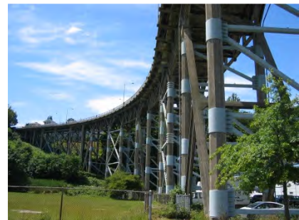
Column bracing at west end of bridge
