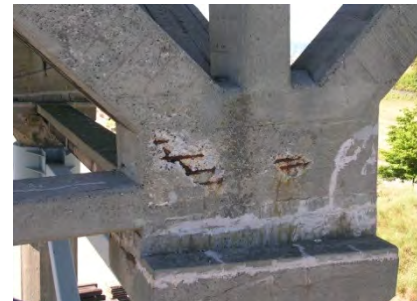
Column bracing at west end of bridge
