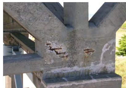
Column bracing at west end of bridge
