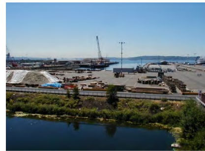
Pier 90 and Pier 91
