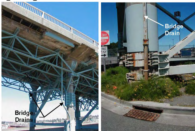
Exhibit 5.10-3 Existing Bridge Drains
