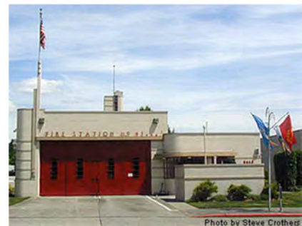
Photo by Steve Crothers Fire Station 41 in Magnolia
