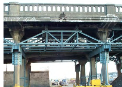
Existing supports and deck repair
