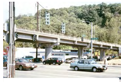
Elliott Avenue West Intersection
