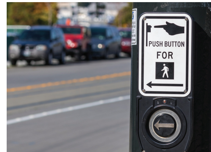
A new signaled crosswalk near 38th Ave SW will increase comfort for people walking
