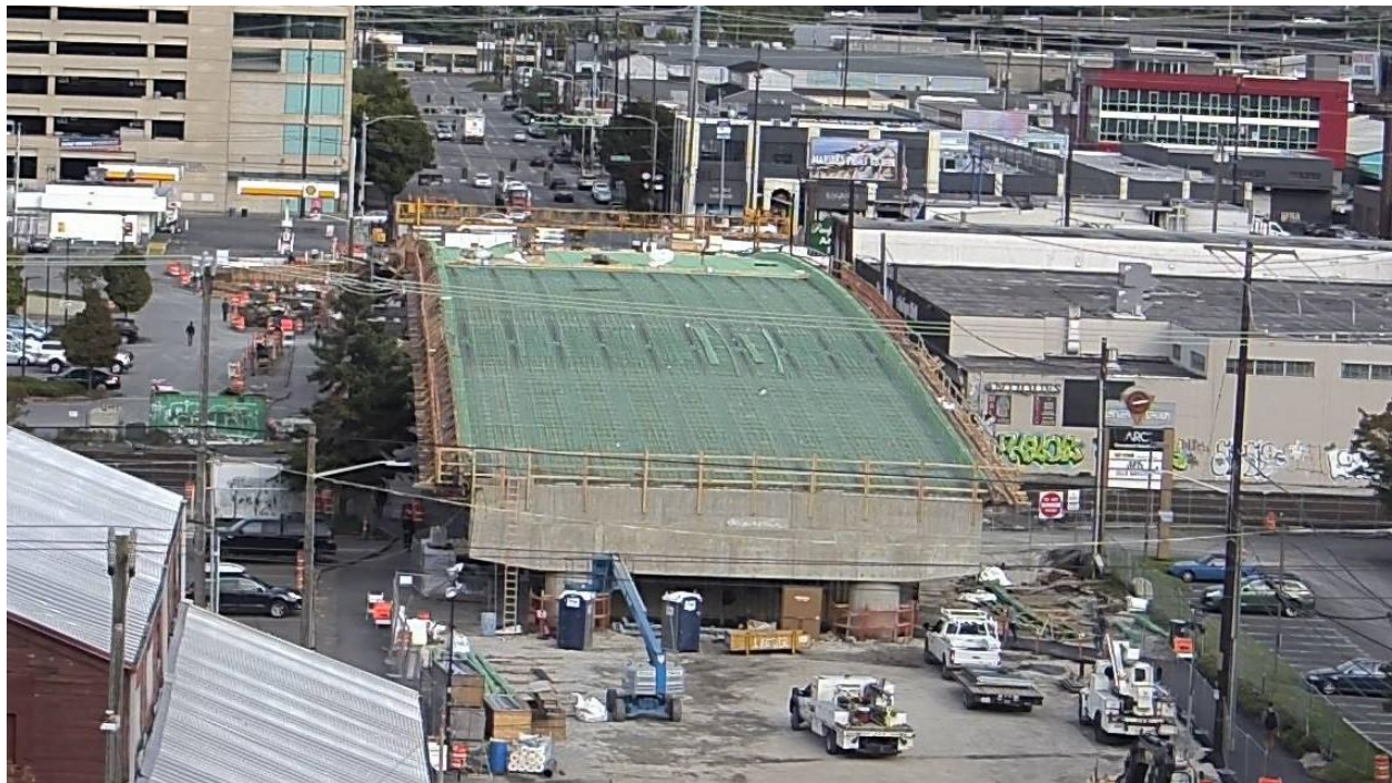
Lander Overpass continues to take shape
