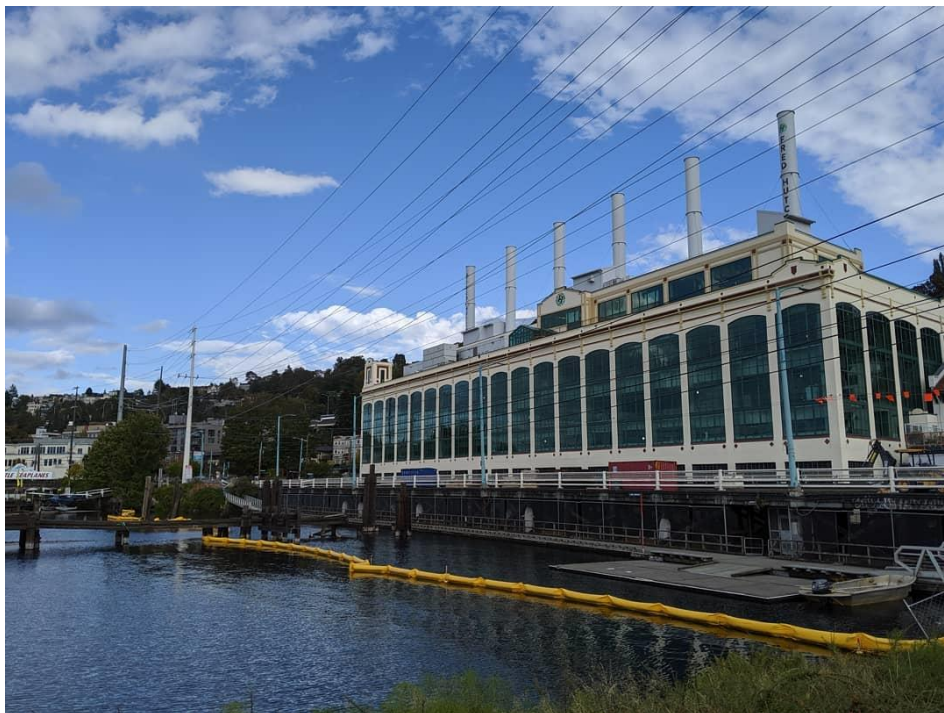
Work begins to replace Fairview Bridge
