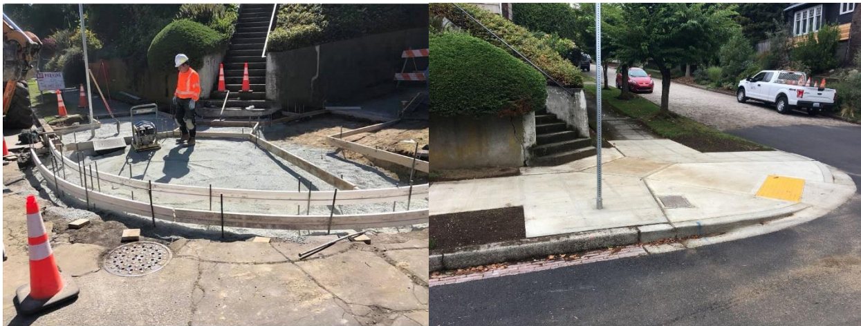
Curb ramp during construction and a completed corner, after construction
