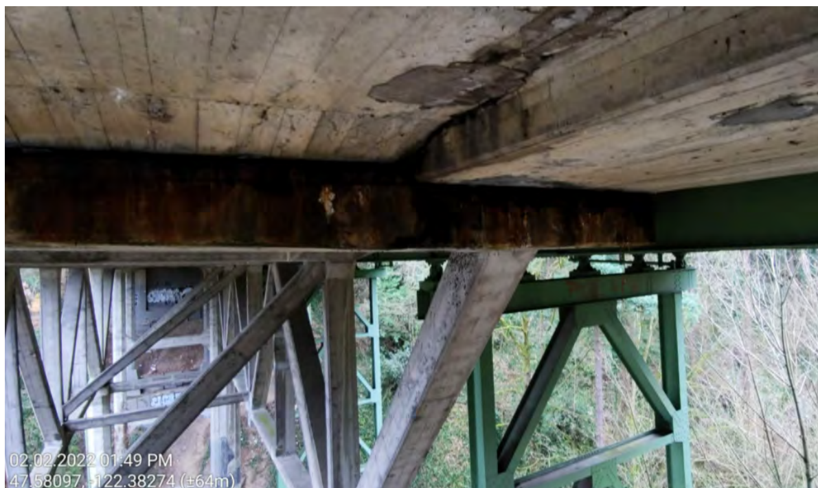
Figure 3.7 Concrete Corbel at End of Concrete Truss (North Bridge, Looking East)
