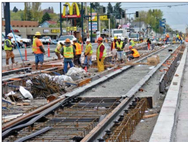
Laying track for Link light rail on Martin Luther King Jr. Way S. at S. Graham St.
