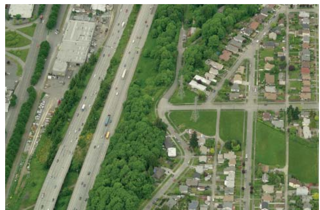
The Chief Sealth Trail has been built in the City Light right-of-way, which is interrupted at ground-level by I-5. Bicyclists need a way to cross I-5 and to connect to the I-90 Trail.
