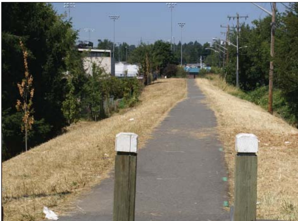
Existing conditions, looking north
