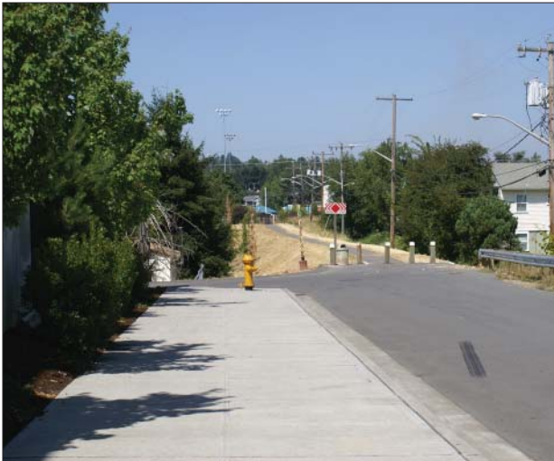
Existing conditions, looking north
