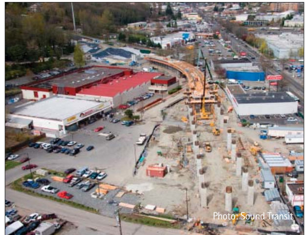
This photo shows early construction activity on the Mt. Baker Station. Light rail will reinforce the transition to a denser, pedestrian-focused urban center.
