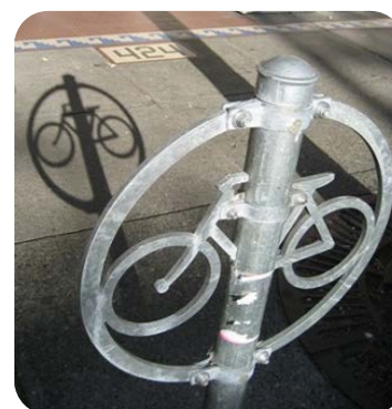
Bicycle Rack Converted from a Meter Pole
