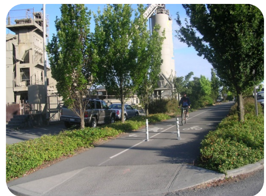
Landscaped Trail in an Industrial Area
