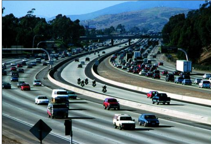
Figure A-3: I-15 Express Lanes in San Diego, CA
