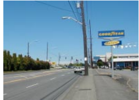
Existing sidewalk conditions along 5th Avenue NE
