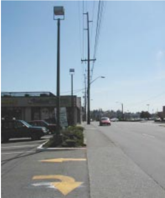
Existing conditions along 5th Avenue NE south of NE Northgate Way
