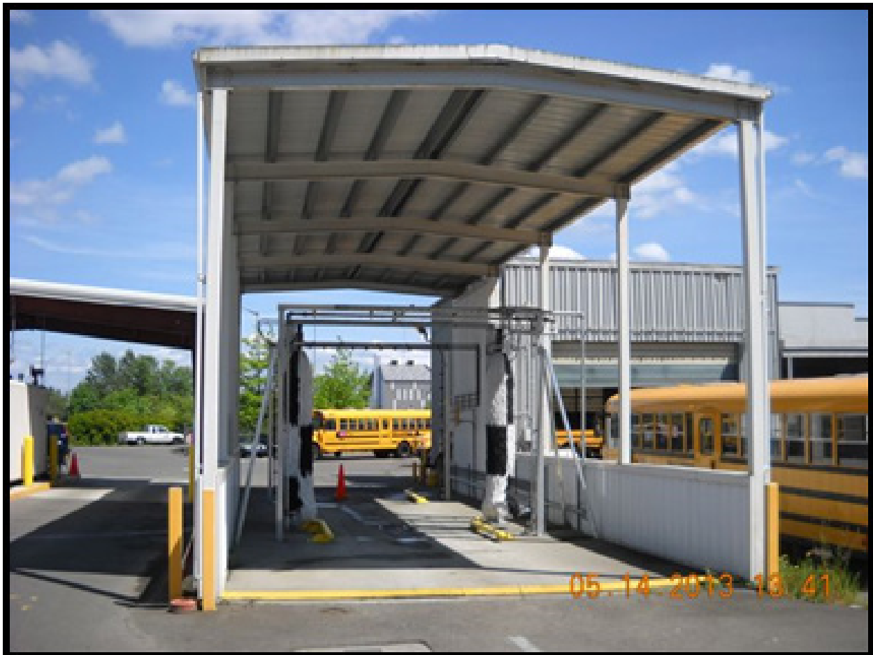
Figure 8. Car Wash Building with Drain to the Sanitary Sewer.
