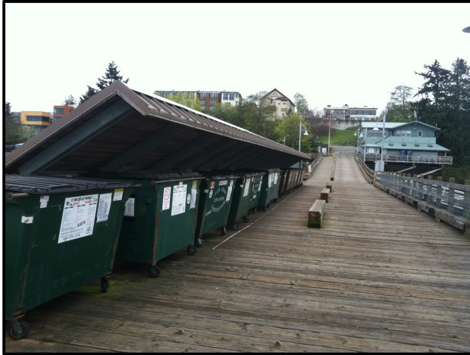
Figure 1. Covered Outdoor Storage of Solid Wastes in Suitable Containers.
