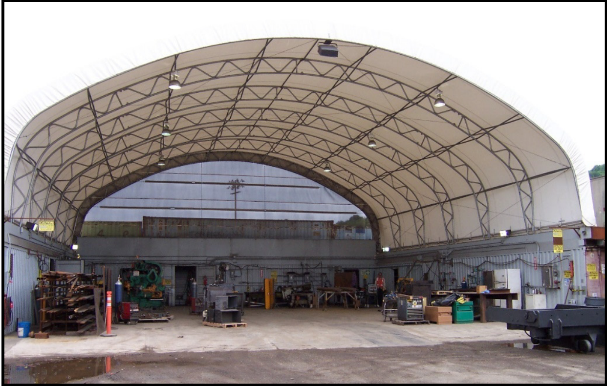
Figure 12. Structure Used to Cover Manufacturing Activities.
