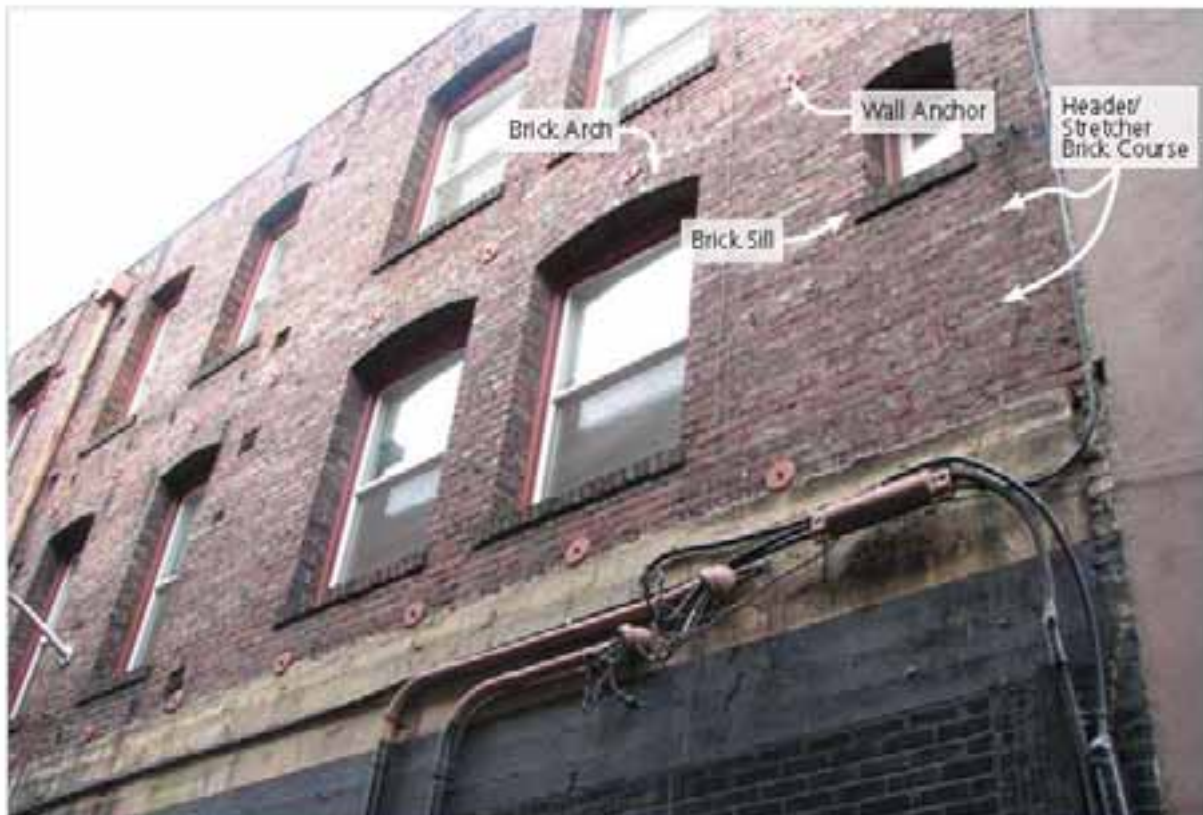
Figure 1. Typical Characteristics of a URM Building.
