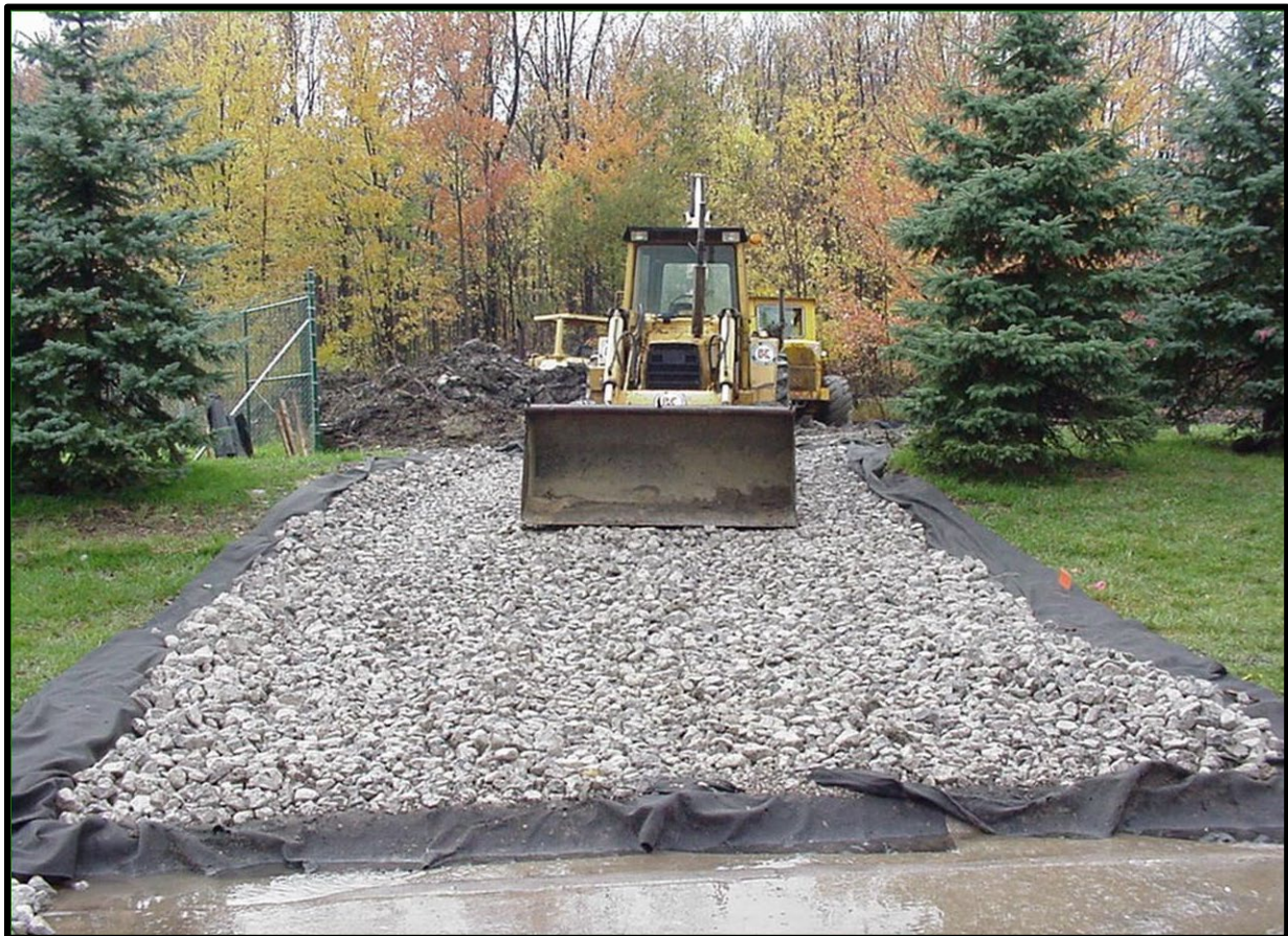
Figure 6. Stabilized Construction Access.
