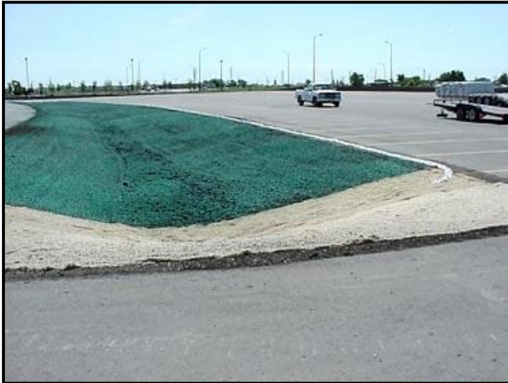
Figure 1. Hydroseeding Method.
