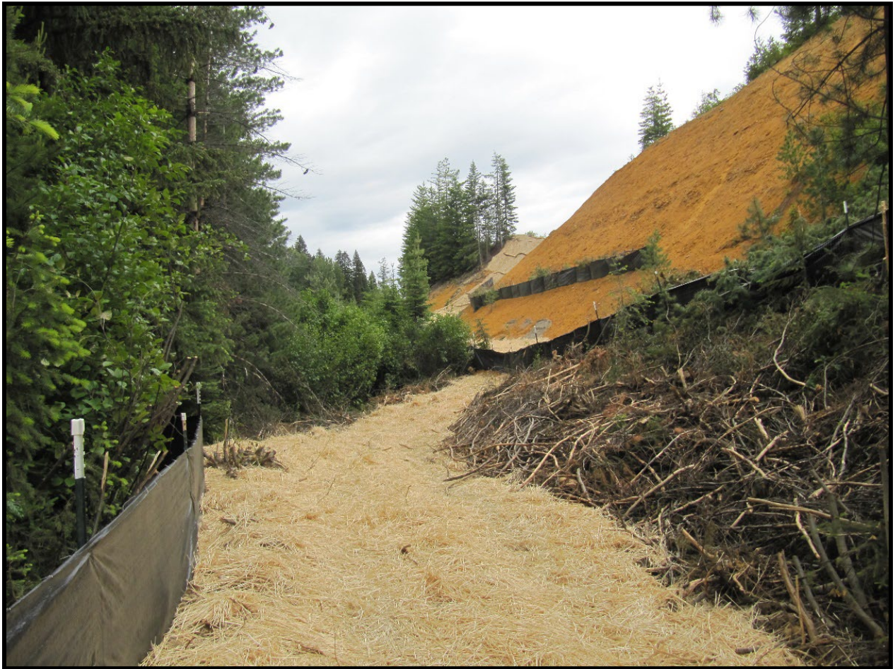
Figure 13. Filter Fence Installed on a Slope.
