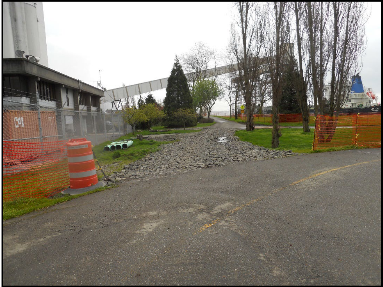
Figure 7. Stabilized Construction Access.
