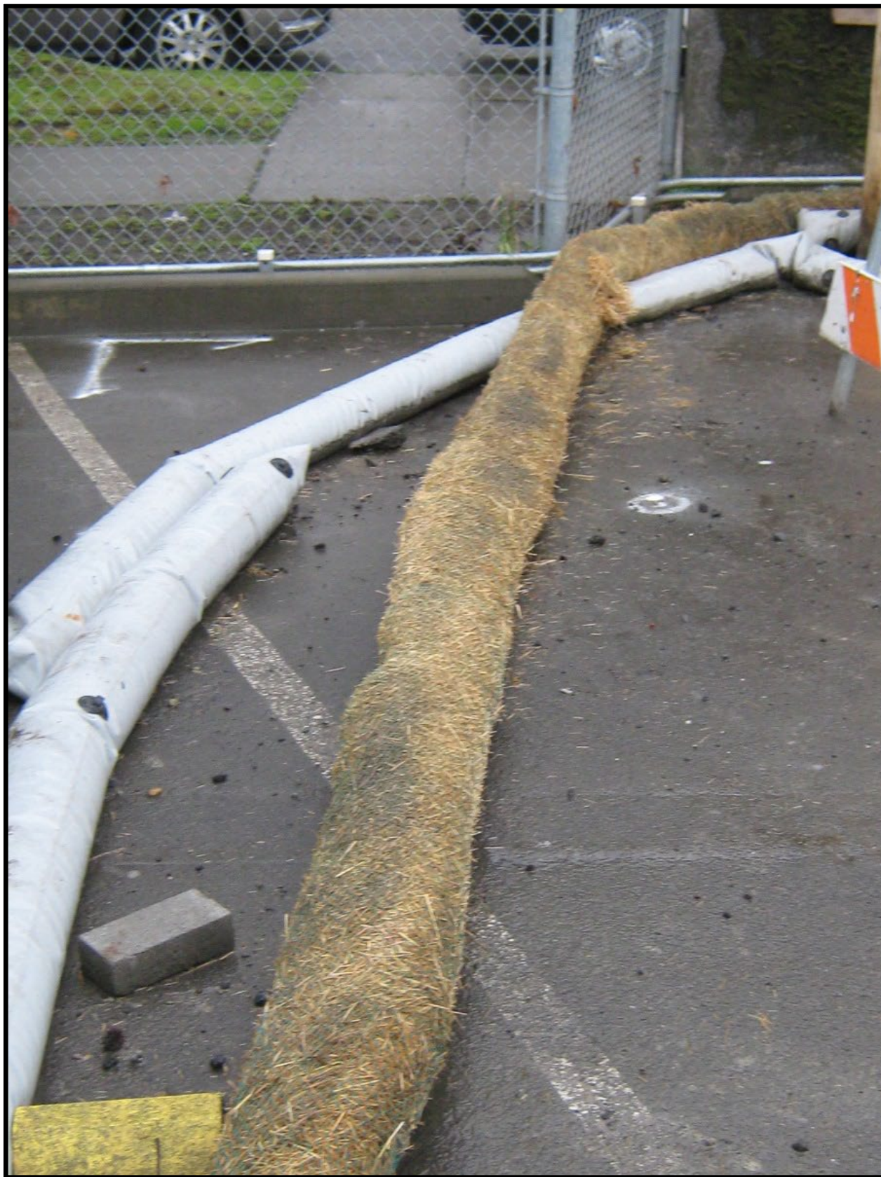
Figure 16. Curb and Gutter Barrier.
