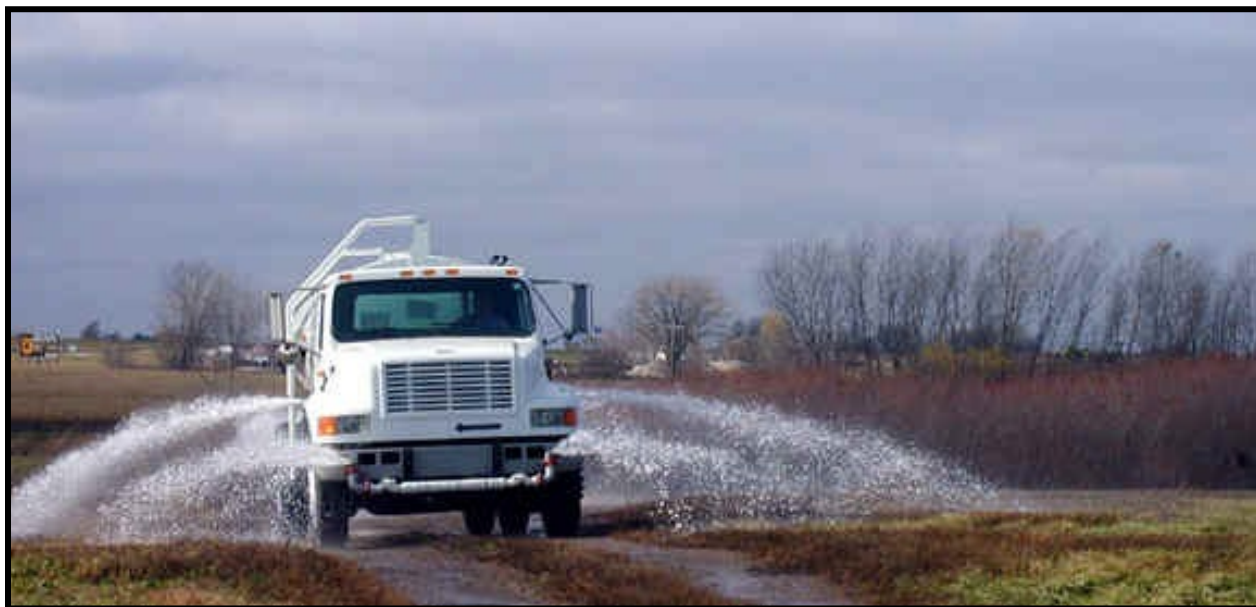
Figure 11. Using a Water Truck for Dust Control.
