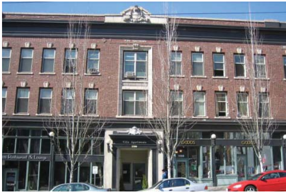
Figure 22a: Villa Apartments
