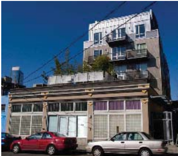
Figure 18: This addition is placed to the rear of the character structure and set well back from the street front, retaining the original proportions, scale and character of the main facade.
