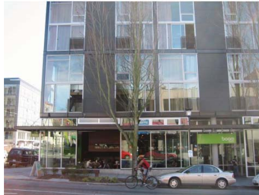
Figure 27: Use of modern materials
