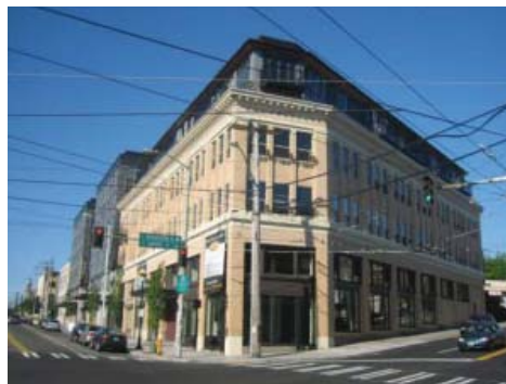
Figure 22f: Trace Lofts
