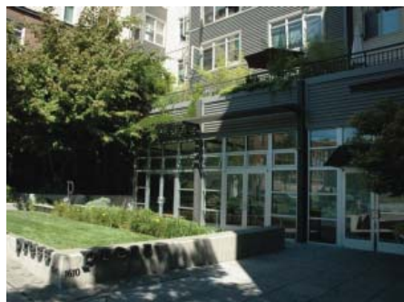
Figure 3: The courtyard of Press Condominiums provides a residential open space amenity on Belmont Avenue E.
