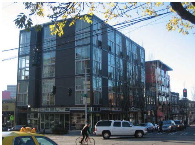
Figure 14: Successful small lot development on Pike Street.
