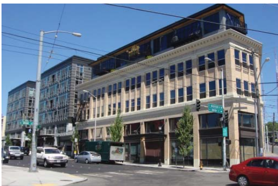
Figure 8: Upper story setbacks maintain street level proportions.
