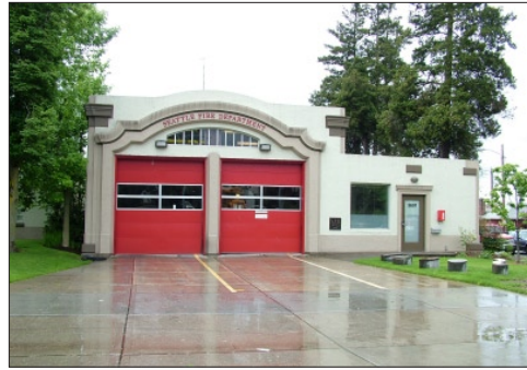
Historic Fire Station 13
