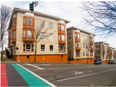
Regular breaks in the building lessen the perceived bulk from the street.
