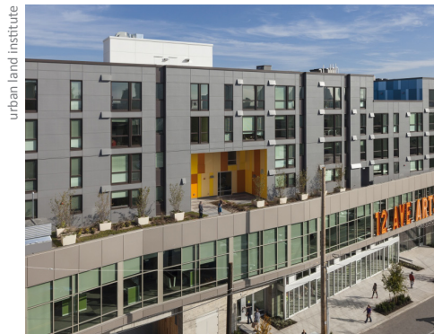
Upper floor setback creates a usable outdoor "community porch" space.
