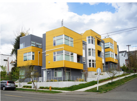
Broken-up building massing avoids a monolithic form.
