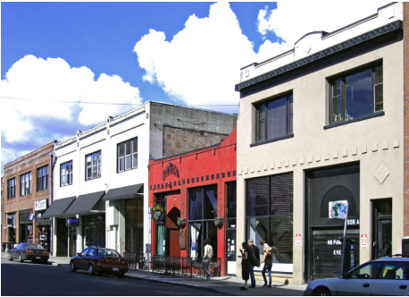
Smaller scaled commercial façades and footprints are conducive to local businesses.
