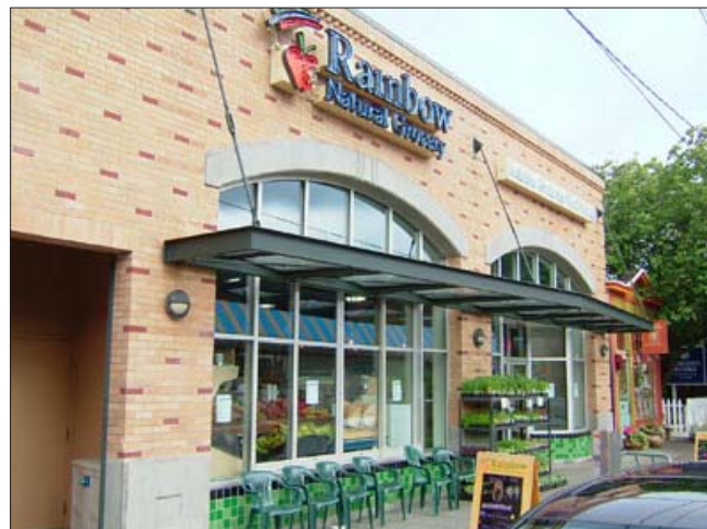
A good example of a storefront that animates the street edge and sustains a pedestrian's interest with a high degree of transparency along the street, through which uses are readily discernable to the passer-by. Overhead cover along the sidewalk and seating adds pedestrian comfort.
