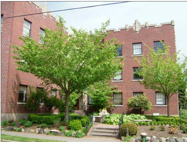
Buildings on corner lots should be oriented to the corner and public street fronts. A prominent, landscaped corner entry can promote visibility at a street intersection, and provides a comfortable place for people.
