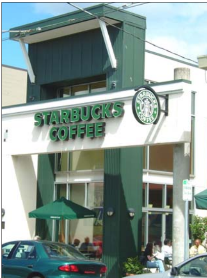
The example above shows metal used as an accent on the exterior of the building, as part of a carefully executed and balanced facade.
