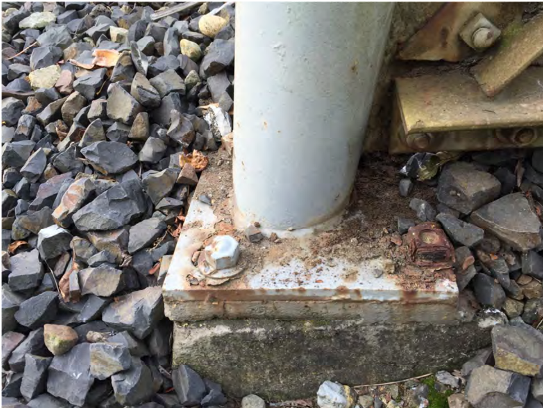
Figure 7 Corrosion at Pier Pipe Base Plate Anchor
