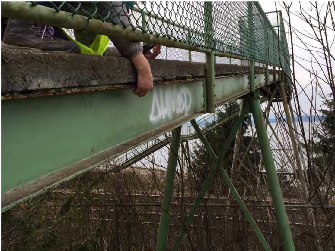
Figure 9 Corrosion at Steel Beam Top Flange
