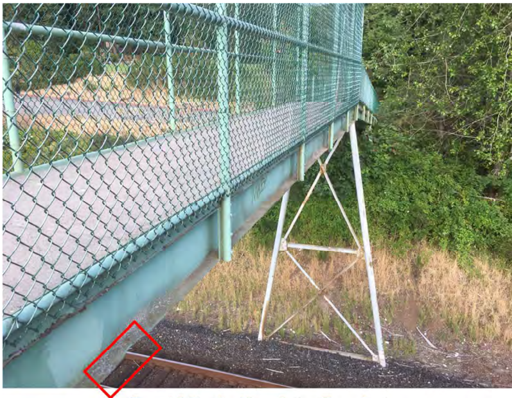
Figure 3 Bridge Steel Beam Bottom Flange Dent
