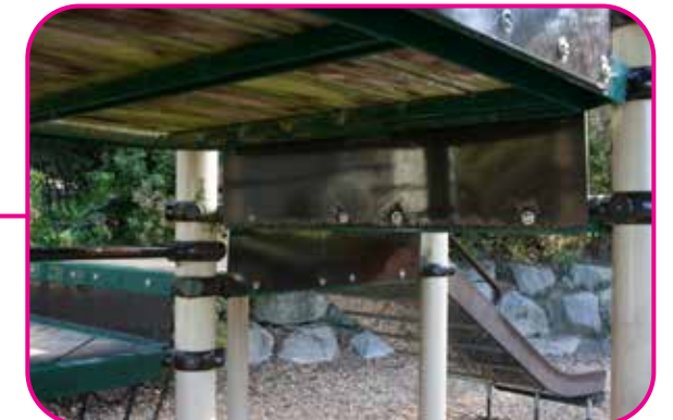
Existing play equipment is in poor condition
