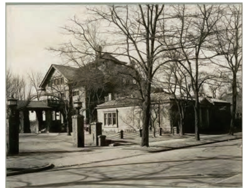
Horace Chapin Henry house, ca. 1935, gallery built in 1917, Carl Gould, Arch. SPL
