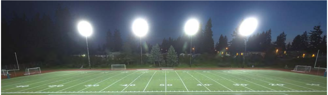
Shielded, Aimable Metal Halide Floodlight System 2015
