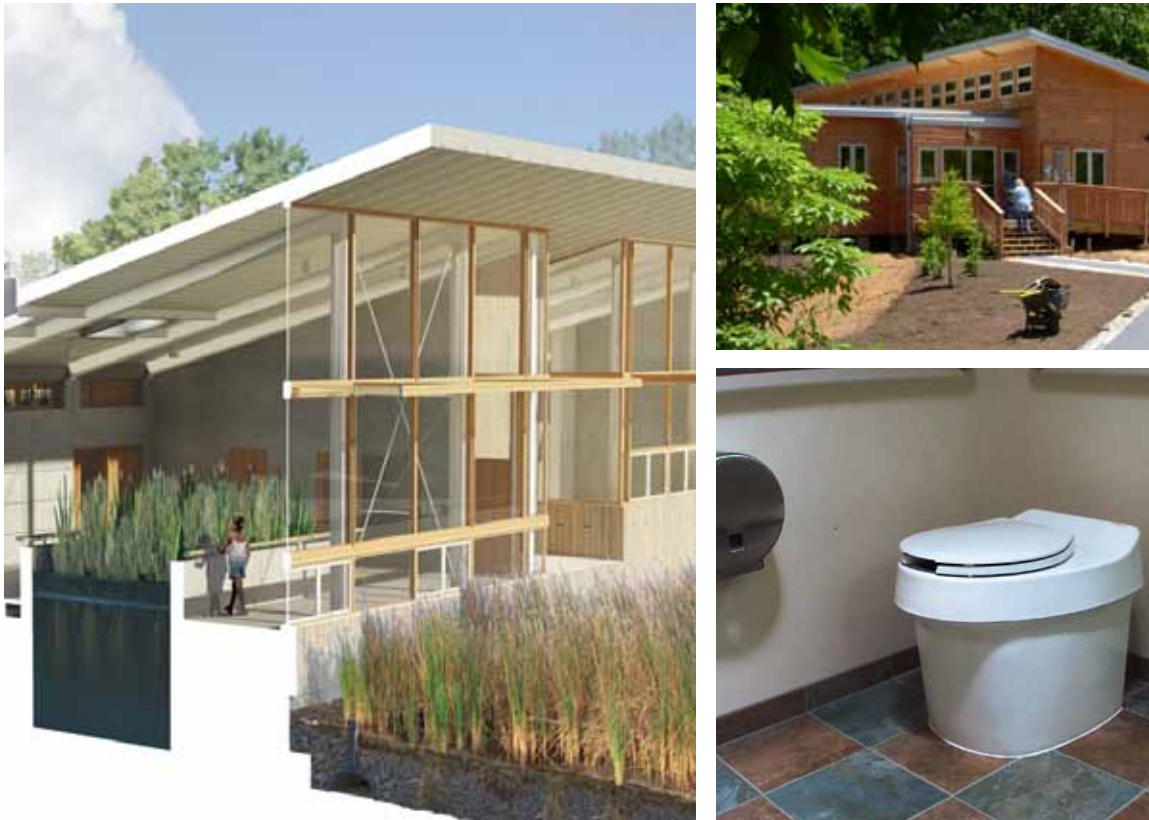
The first two certified Living Buildings in the United States, The Omega Center for Sustainable Living in Rhinebeck, NY (above left) and Tyson Research Center’s Living Learning Center in Eureka, MO (above right) utilize different strategies to manage water and waste on-site. The Omega Center collects wastewater from the surrounding campus and treats it on-site through an eco-machine and constructed wetlands. Tyson’s potable water is provided by a chemical-free rainwater harvesting system. The project includes composting toilets and a sub-surface constructed wetland to treat greywater. Images courtesy of BNIM Architects and Clivus Multrum.
