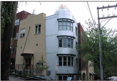
A corner building form that demarcates an important gateway/street corner.
