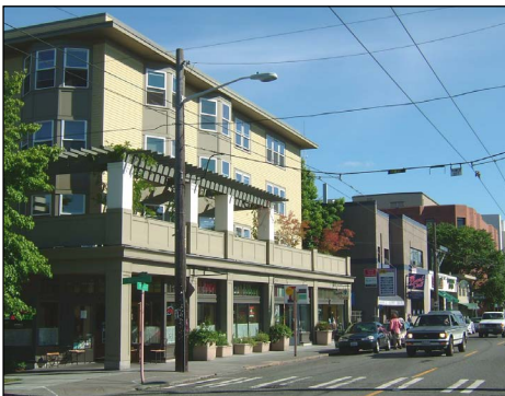
Landscaping softens the setback from the ground level retail to residential levels above.
