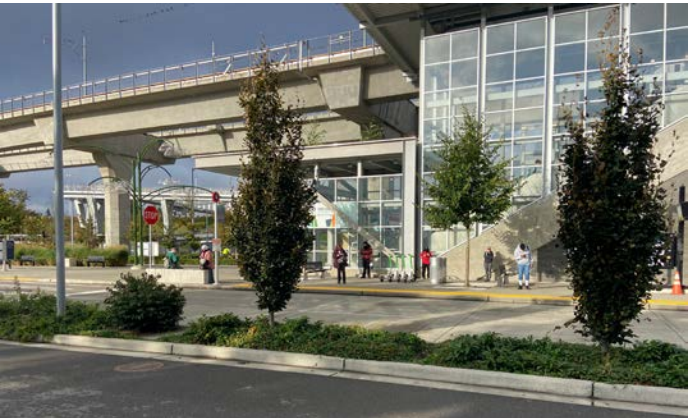
Top: The John Lewis Memorial Bridge represents a long-term investment in Northgate’s transformation toward becoming a walkable, transit-oriented community. Above: E-scooter rentals are lined up at the light rail station, helping transit riders make their nearby connections without a car.
