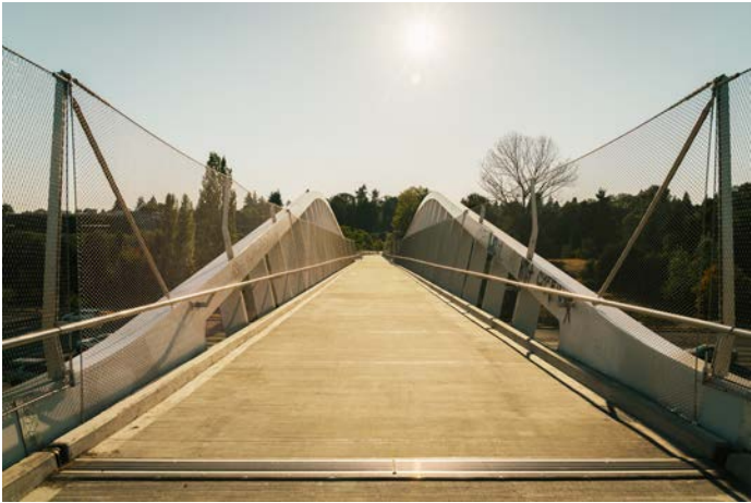
The John Lewis Memorial Pedestrian Bridge is particularly exposed to the elements.
