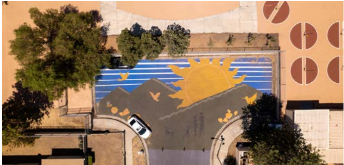
Cool pavements have been implemented in many LA neighborhoods, with priority given to areas most frequented by children and seniors. A year after these cool pavements were introduced, researchers found a 10-degree reduction in surface temperature and 2-degree reduction in ambient temperature on hot days. Image: NBCU Academy.
