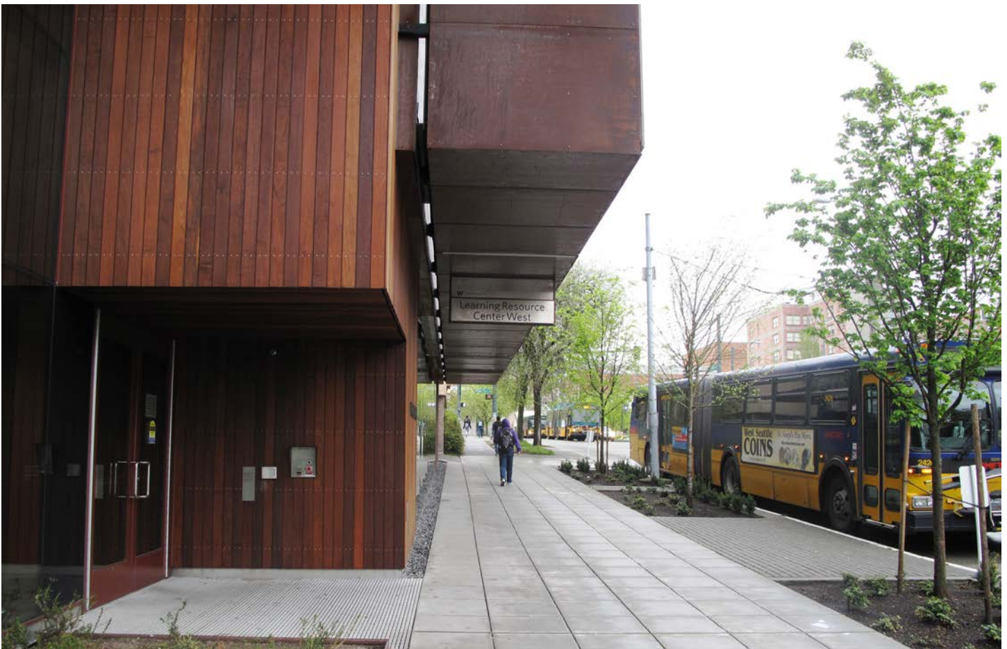
New student housing along Campus Parkway
