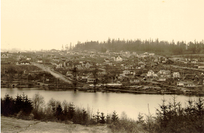
Asahel Curtis, University District, 1905. The University campus is in the trees at the back.
