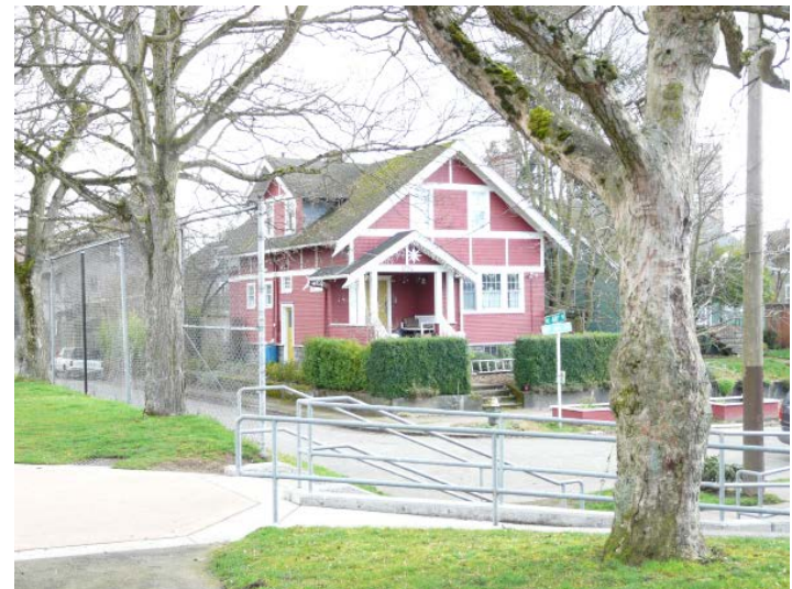
Example of single-family structures located within ten-minute walk of the future station
