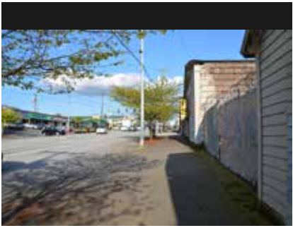
A cluster of dilapidated buildings covered in graffiti makes the neighborhood appear unsafe
