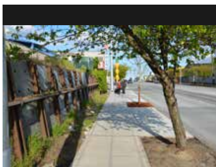
A long, blank, retaining wall attracts graffiti and trash, discourages visitors from continuing on.
