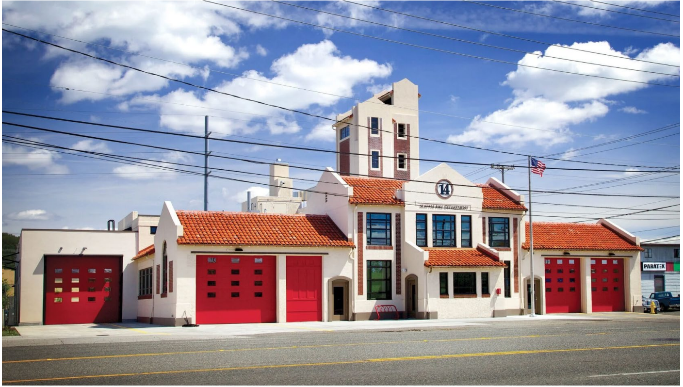
Seattle Fire Station 14 serves the Duwamish MIC
