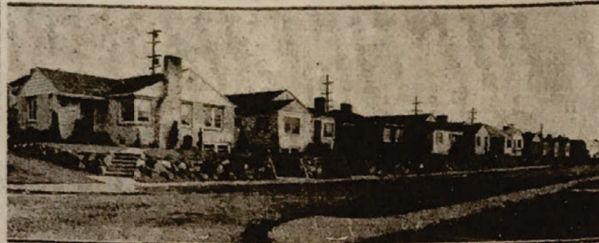
This row of new homes, part of those built by Earl F. Mench during 1939, will be duplicated several times in 1940 as the prominent builder speeds his production of low and moderate-cost residences. Starting with a preliminary group of twenty properties, Mench expects to build fifty new homes. Homes shown here range in price from $2,000 upward, but this year's production will include properties priced as low as $2,800.
