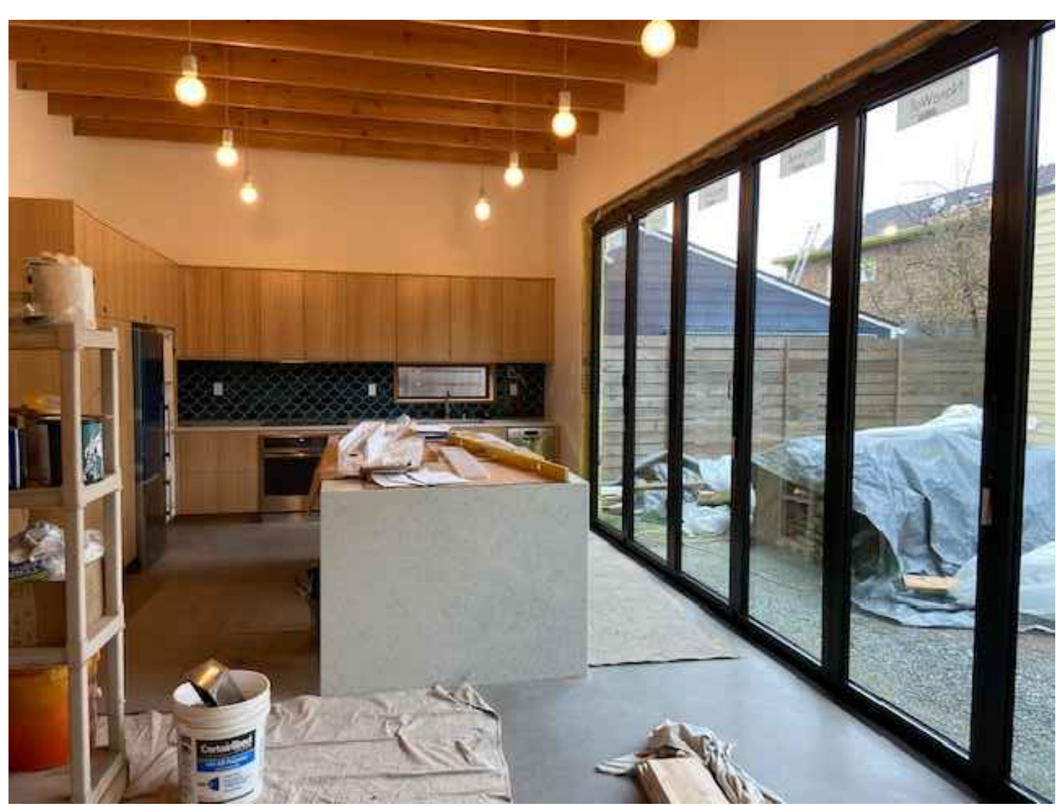
VARIANT UNDER CONSTRUCTION WITH ALTERNATE OPENINGS AT LIVING/KITCHEN
