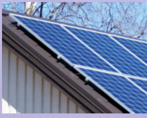
SOLAR PANELS ON METAL ROOF
