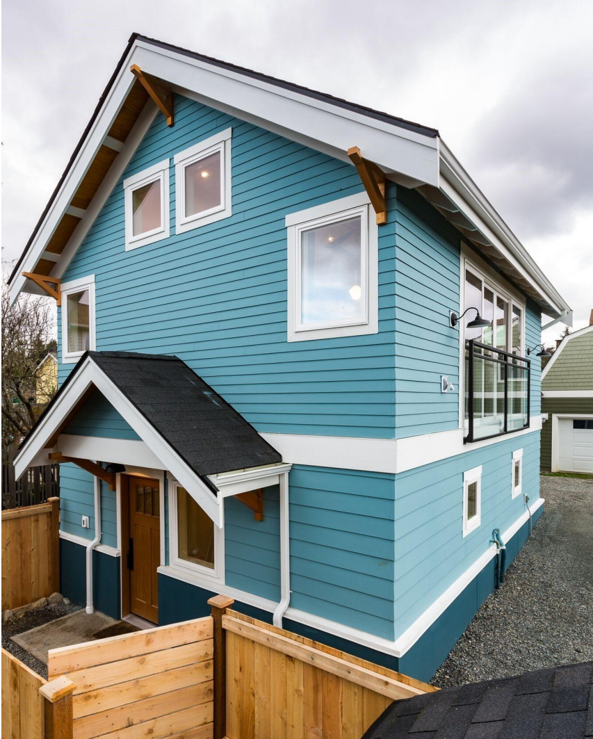
DADU entry and south facing Juliette balcony.
