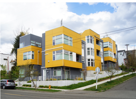
Broken-up building massing avoids a monolithic form.
