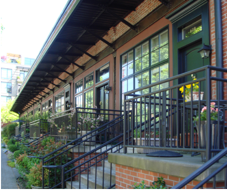
Raised entries creating a private stoop at residential entrances.
