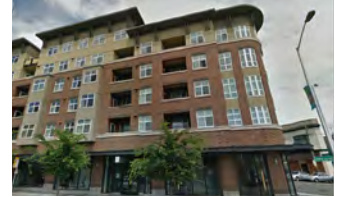
Typical new building with ground level commercial and residential uses above.
