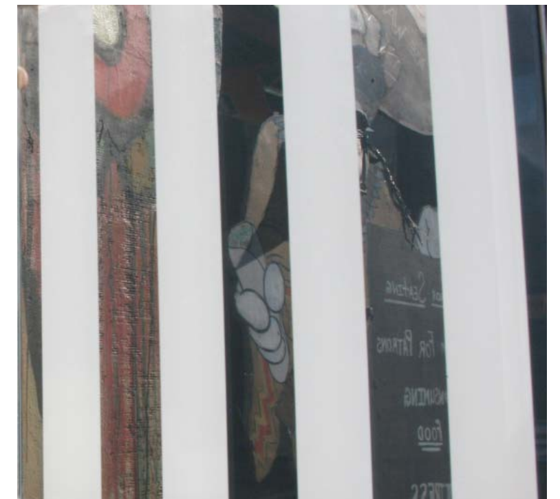
San Francisco Planning Department - Standards for Bird Safe Buildings: -1/4" wide strips @ 4" spacing qualify as bird-safe
