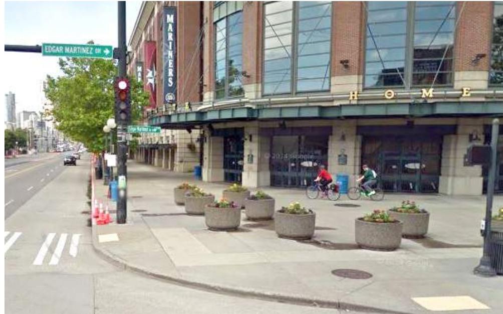
1st Ave S // Looking North
