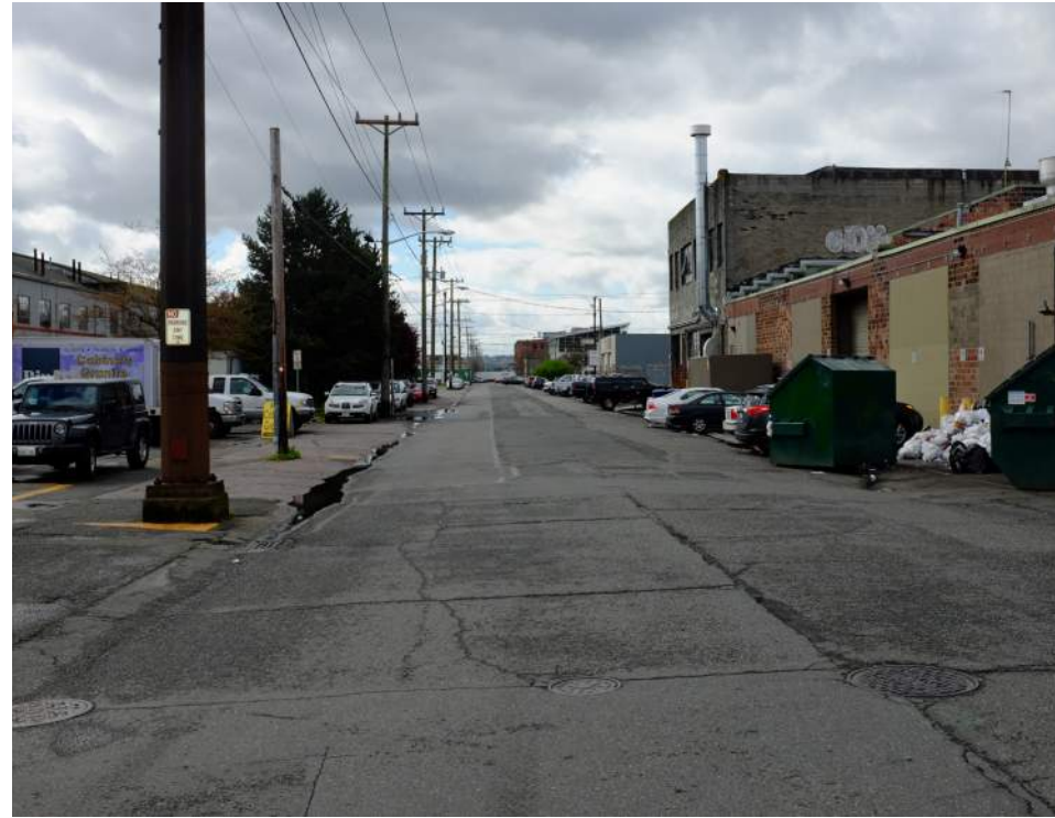
Looking South From S. Massachusetts St.
