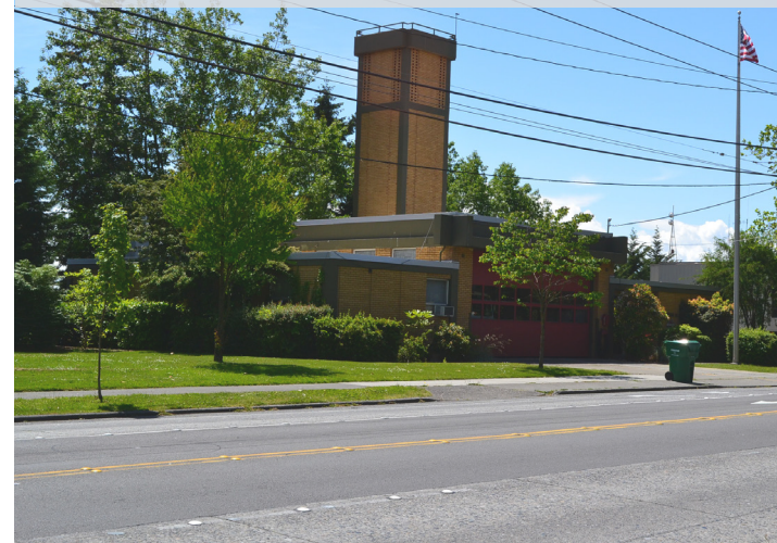
Looking southwest along E. Roanoke St.
