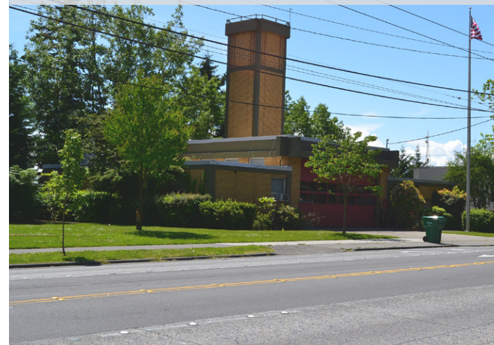
Looking southwest along E. Roanoke St.
