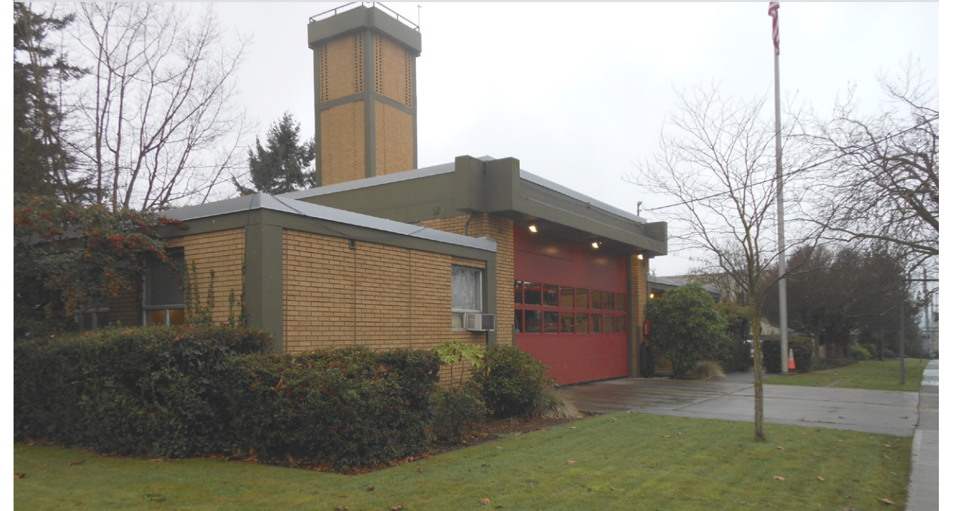
Existing Fire Station 22, December 2013.
